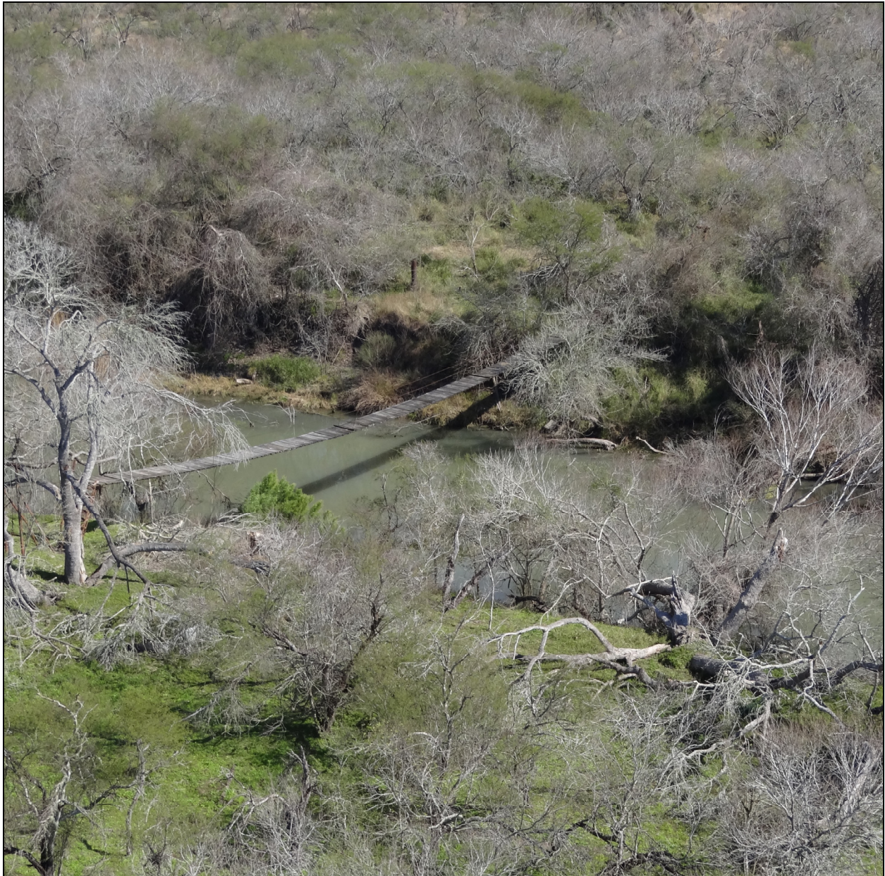
Figure 5.15: Cable Bridge in East Riverside Well Field
