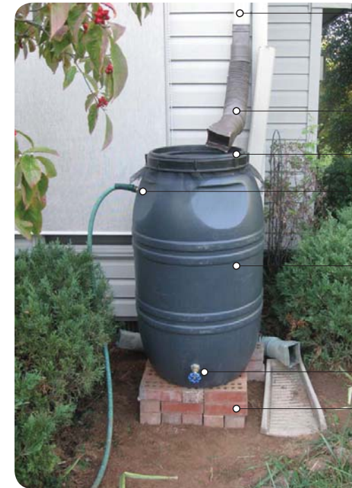
Example of a residential rainwater harvesting system
