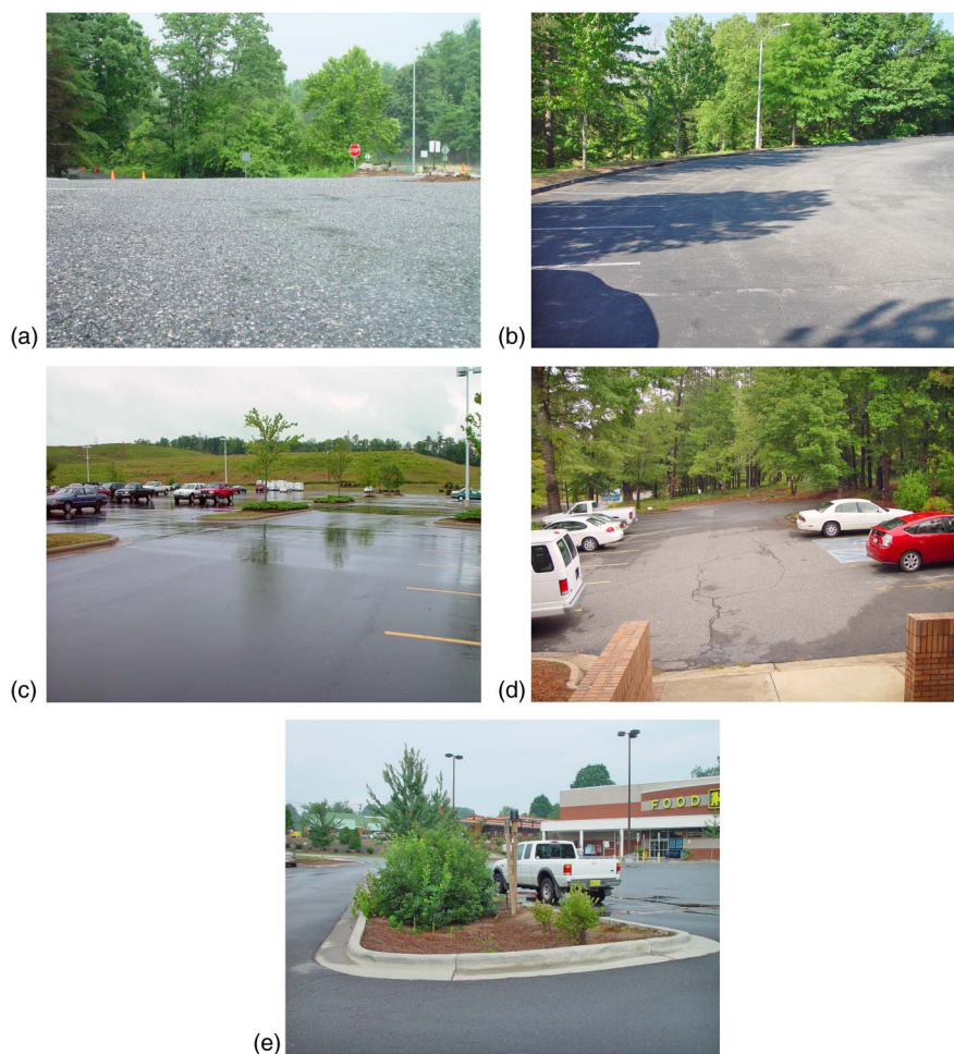
Fig. 1. Contributing catchments: (a) Asheville chip seal site; (b) Asheville hot-mix asphalt site; (c) Lenoir full sun site; (d) Lenoir shade site; (e) Brevard bioretention areas
