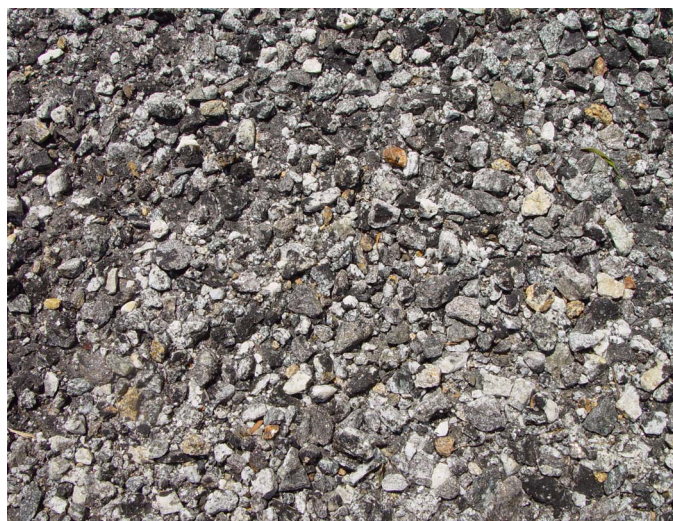
Fig. 2. Light-colored chip seal applied to the pavement surface
