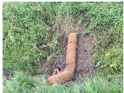
FIGURE 4: FILTER SOCK AT THE END OF A TREATMENT PRACTICE
