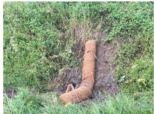
FIGURE 4: FILTER SOCK AT THE END OF A RETROFIT
