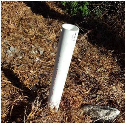
FIGURE 3: PVC MONITORING WELL
