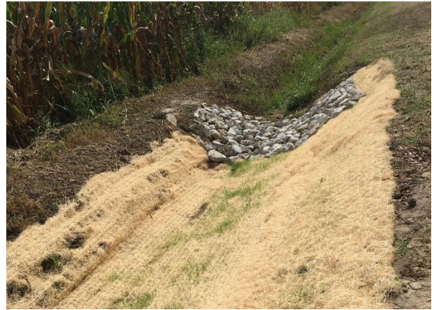
FIGURE 5: INLET PROTECTION AND EROSION CONTROL MATTING (CURLEX®)
