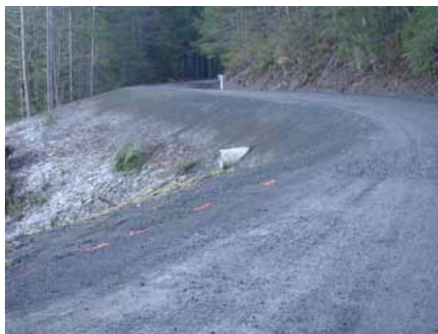
FIGURE 38 Deep patch during and after construction in Gifford Pinchot National Forest in Washington (Courtesy: B. Collins).
