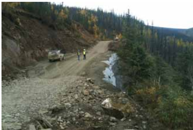
FIGURE 37 Early work by a contractor creating a geotextile wall in Alaska, and geotextile wall on fill slope of road in Klamath National Forest in California (Courtesy: J. Currey and G. Keller).
