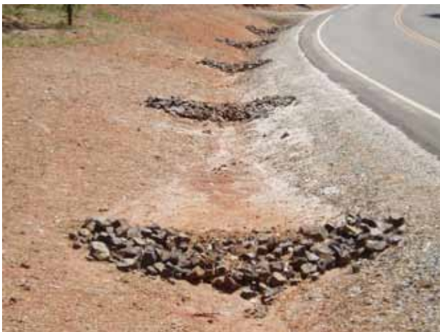
FIGURE 21 Rock pile check dams (Courtesy: G. Keller).
