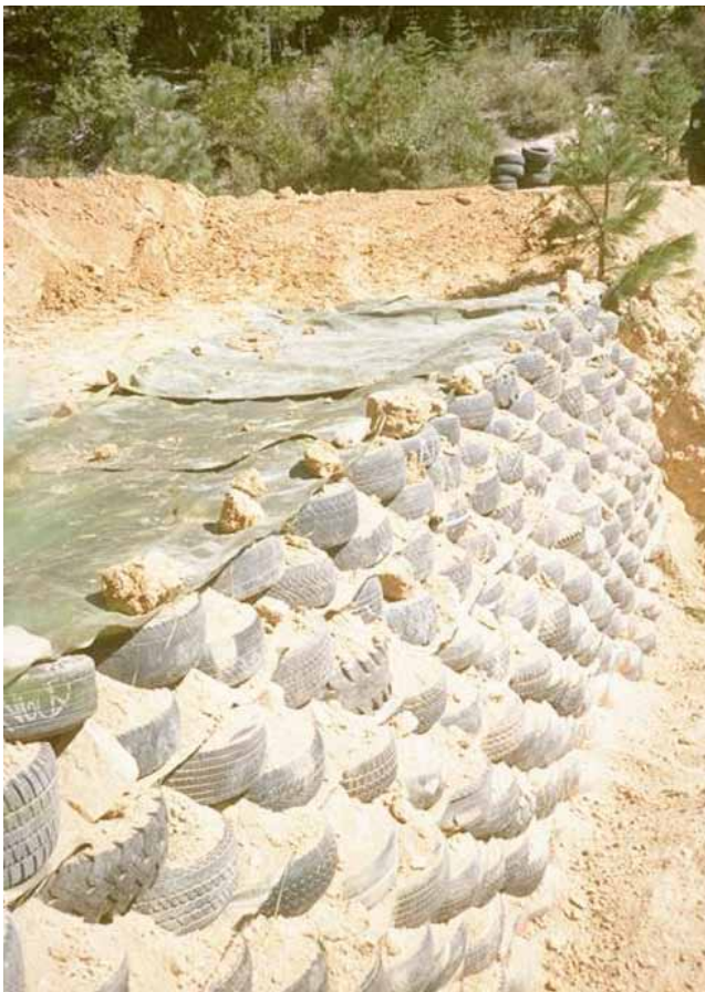
FIGURE 39 Tire wall and construction (Courtesy: G. Keller).
