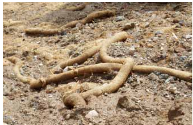
FIGURE 22 A successful application of wattles on a stable cut slope (left); A failed application of wattles that were placed over an unstable, over-steep fill slope (right) (Courtesy: G. Keller).
