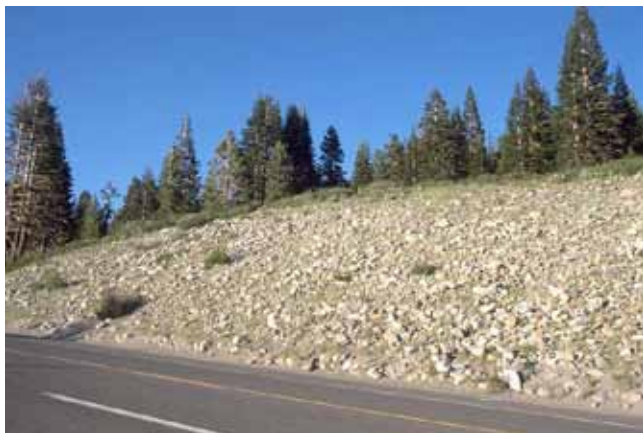
FIGURE 18 Rock blanket on a cut slope for erosion control, Lake Tahoe (Courtesy: G. Keller).
