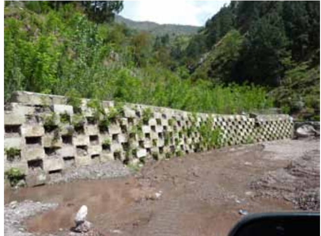
FIGURE 29 Post-earthquake (2005) slope stabilization using a masonry crib wall and layered planting of native trees and bushes, Balakot-Kaghan Road (N-15), Pakistan (Courtesy: A. Faiz).
