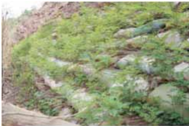
FIGURE 31 Vegetated soft gabion wall (Shah 2008).
