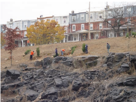
Large holes are hand dug for balled and burlapped Eastern red cedars.
