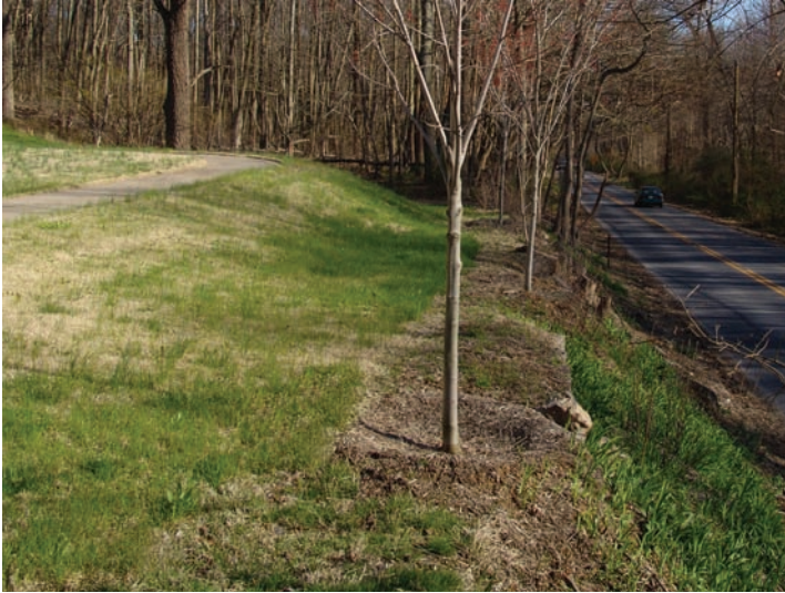
Semi-circular mulch barriers at the base of these red maples capture rainwater from the upper slope and direct it to the root area where it can slowly infiltrate.
