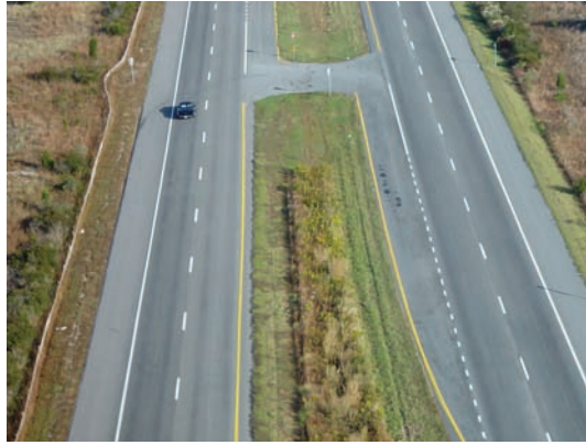
Edges of crossovers are mowed to allow visibility for turning vehicles.
