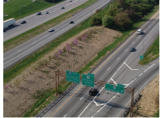
The berm between I95 and 495 has been planted with trees, shrubs and warm-season grasses. Mowing is routinely required at the base of the berm only and warm-season grasses are cut back once each year.
