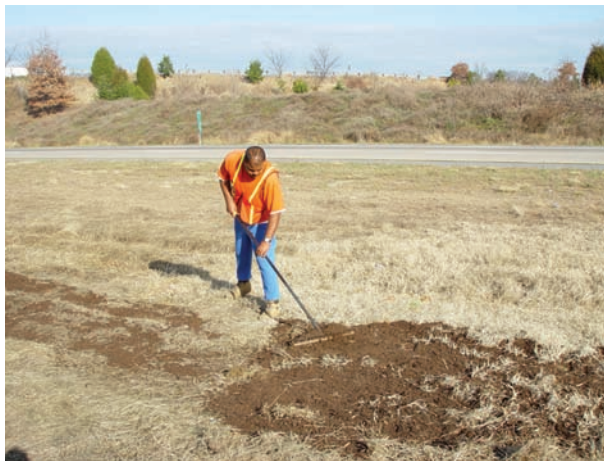
For small areas, seed is mixed with a moist carrier and spread using a wheelbarrow and hard rake.
