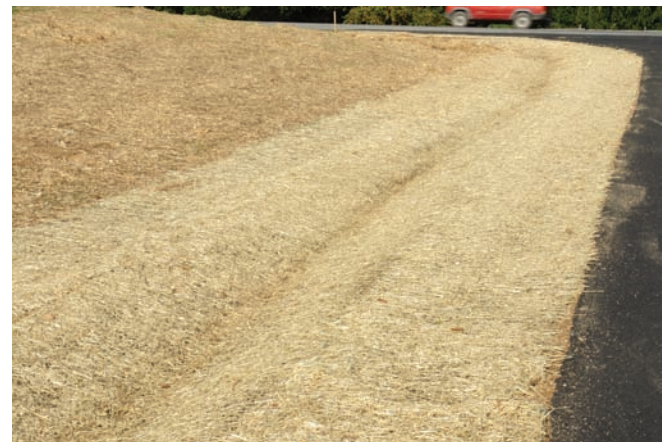
A fiber blanket lines this ditch on a newly constructed roadside.
