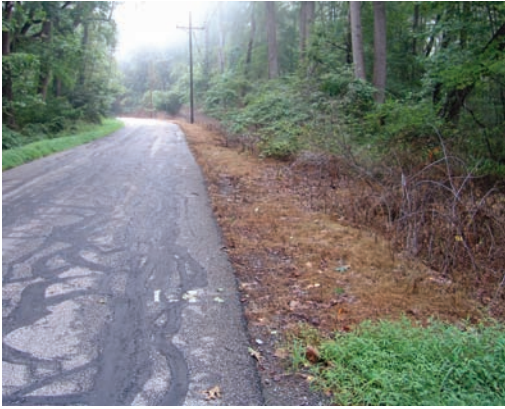
A directed spray of glyphosate was used to control Japanese stilt grass and other weeds on the roadside edge.
