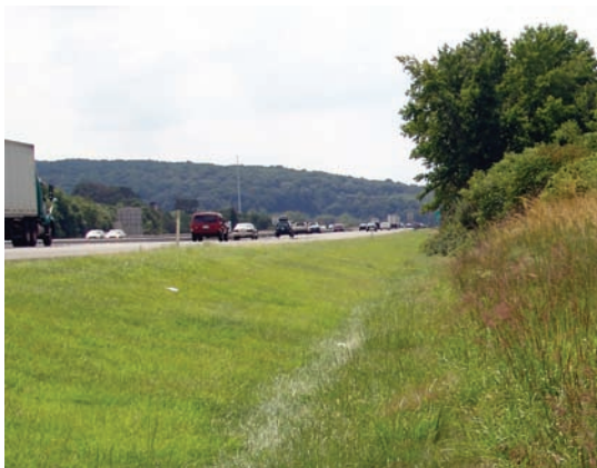
Along I95, the roadside is mowed one mower pass beyond the swale.
