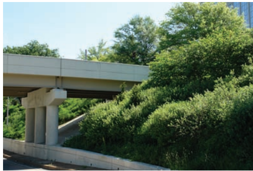
The deep, spreading roots of colonizing shrubs like sumac stabilize even a steep slope.
