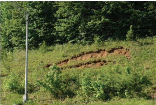
This cool-season grass mixture is not deeply rooted enough to prevent erosion.
