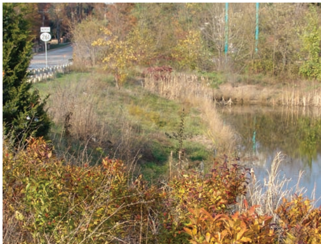
Mowed turf is restricted to a narrow strip adjacent to the guardrail. The slope is planted with grasses and other low maintenance vegetation and serves as a buffer enhancing the habitat quality of this stormwater pond.
