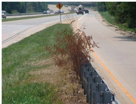
Herbicides are used to control tall vegetation obstructing the guard rail.
