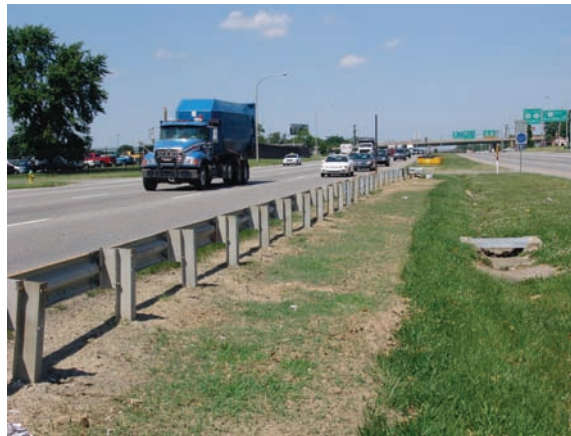
Low fescue seeded under guard rail provides a low cover that stabilizes soil but requires only infrequent mowing.
