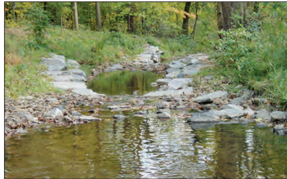
Wing deflectors in Stony Run in Baltimore, Maryland, are used to redirect flow in the stream to concentrate flow away from the banks and toward the center of the stream.
