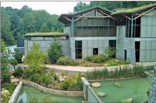
Routing water from a green roof through a series of ponds can reduce runoff from the building's roof and also can provide a green space for enjoyment.
