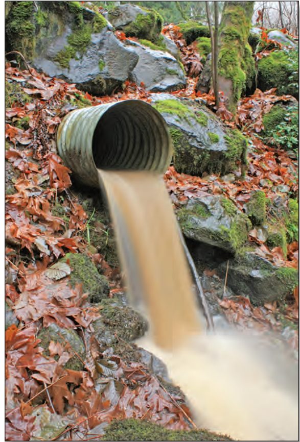
Figure 4. Water-quality sampling at stormwater outfalls, such as this one in Rock Creek, Oregon, has determined that runoff from urban areas contains an array of pollutants that are harmful to aquatic life.
