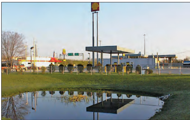
Figure 7. Traditional stormwater management focused on the use of large ponds to reduce the peak rate of stormwater flow and sediment concentrations. Photograph from Center for Watershed Protection.
