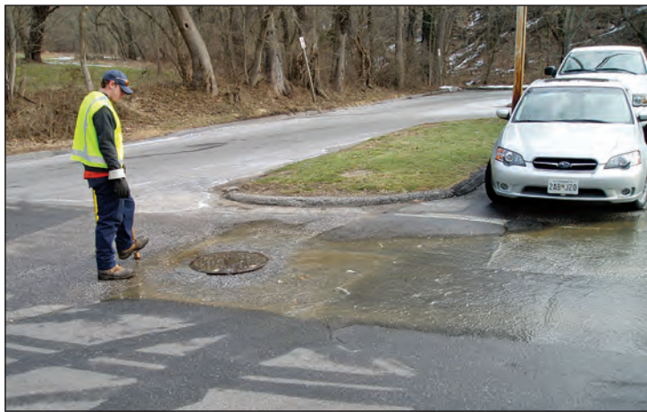
Figure 27. Sanitary sewer overflows can be caused by clogs in the sanitary sewer system or by infiltration of groundwater into the system through cracks in deteriorating pipes. This sanitary sewer overflow in Ellicott City, Maryland, discharged untreated wastewater into a parking lot before maintenance crews were able to fix the problem. Photograph from Center for Watershed Protection.
