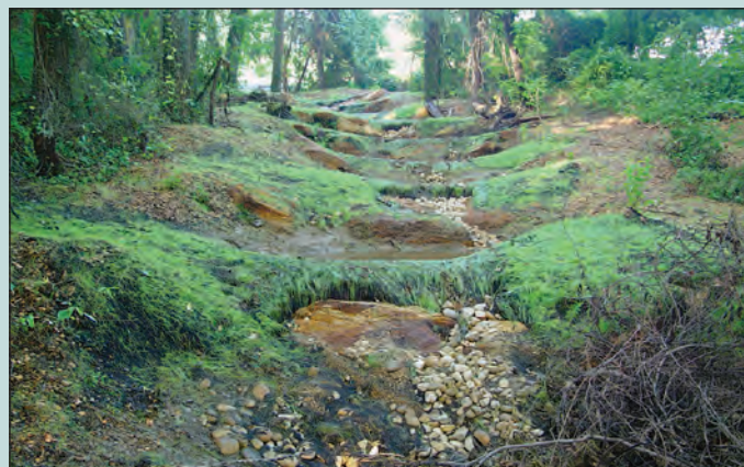
Figure 30. Regenerative Stormwater Conveyance System in Anne Arundel County, Maryland. Photograph by Keith Underwood, Underwood & Associates.
