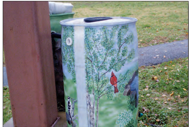
Routing water from downspouts into rain barrels can reduce the amount of runoff diverted to storm drains and provide a significant source of water for lawn and gardens during the summer.
