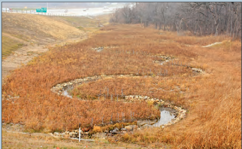
Figure 6. Stream restoration project on an unnamed tributary to the Root River, Wisconsin. This formerly dry ditch in a major interstate interchange now provides diverse intermittent pool habitat for birds, insects, amphibians, and reptiles during dry spells. A 400-foot culvert under the road is designed to allow fish passage to headwater areas during runoff.
