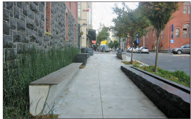
Figure 16. Portland, Oregon, incorporates sustainability principles and practices into the city’s land-use planning. One of these practices is known as a Green Street, which is a vegetated facility that manages stormwater runoff at its source. In the photograph above, water from the street is diverted into a vegetated planter in the sidewalk. Photograph from Center for Watershed for Protection.
