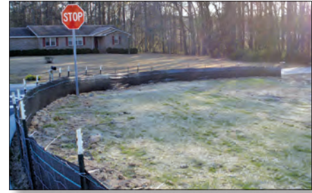
Silt fences are used to contain sediment on a development site.
