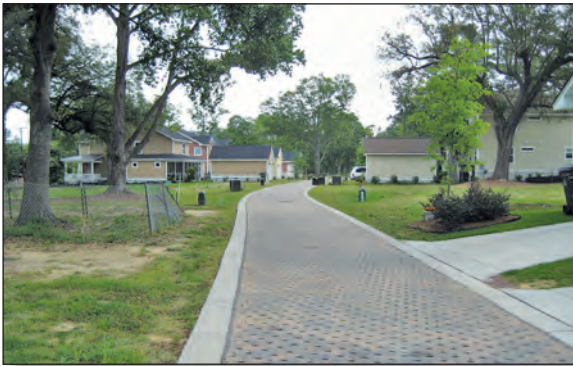
This Richland County, South Carolina, street uses permeable pavers that allow rainwater to infiltrate instead of generating excessive runoff.
