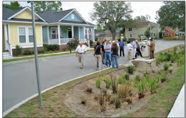
Vegetated swale in the Noisette subdivision in Charleston, South Carolina, is designed to reduce runoff from the roadway.
