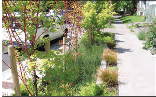
Figure 33. A green street in Portland, Oregon, a previously impervious street surface that was transformed into a landscaped green space that captures stormwater runoff and uses plants and soil to filter pollutants. Photograph from Center for Watershed Protection.
