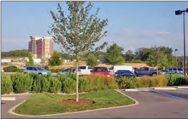
Rain garden/bioretention in a parking lot.
