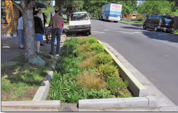
This curb extension bioretention in Portland, Oregon, collects and removes pollutants from runoff and also serves as a traffic calming device.
