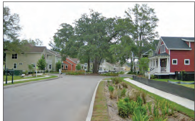
Figure 8. Low-impact development (LID) is a more recent approach to stormwater management that uses site design to reduce runoff and conserve natural areas and incorporate smaller stormwater practices that are distributed throughout a site. This development in Charleston, South Carolina, includes several LID features, including open space preservation and the use of vegetated swales to convey and treat road runoff. Photograph from Center for Watershed Protection.
