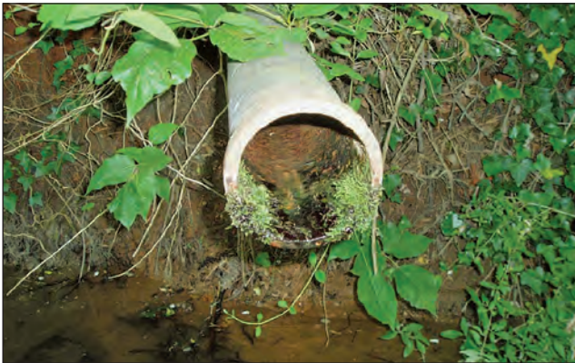
Figure 37. Algae growth on this stormwater outfall is an indicator of the presence of sewage. Flows of sewage to the storm sewer system enter local streams untreated and are considered an illicit discharge.
