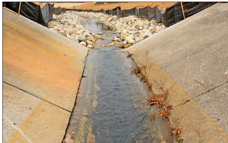
Figure 5. This concrete channel in Villamann Creek, Wisconsin, is designed to quickly transport water downstream to reduce local flooding and protect infrastructure. Just upstream, the concrete channel was recently removed and a flood plain was created to provide more flood attenuation, habitat diversity, and beauty for stream and flood-plain organisms, including humans.
