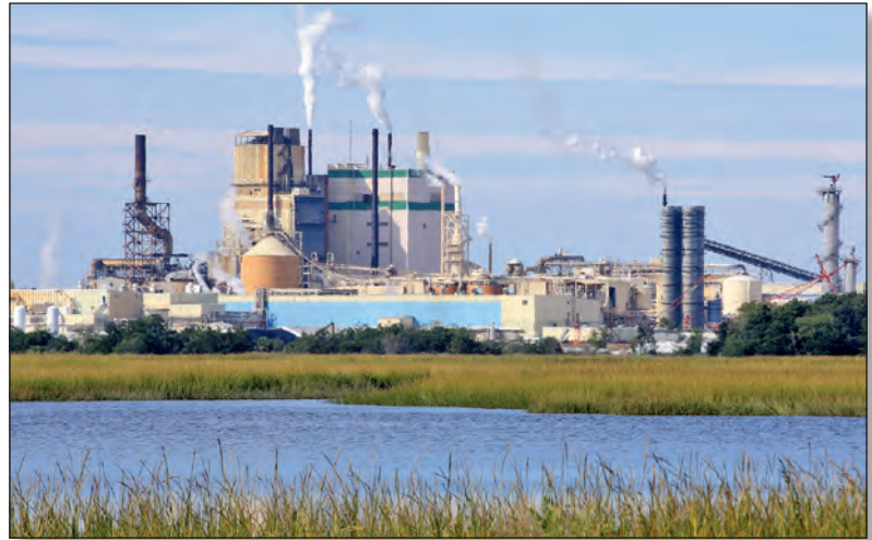
Figure 3. Discharges of waste from industries into nearby waterways was once a common practice prior to regulated permitting under the Clean Water Act.
