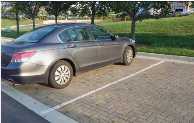
Permeable pavements are used in low-traffic areas to promote runoff reduction by infiltrating rainwater.
