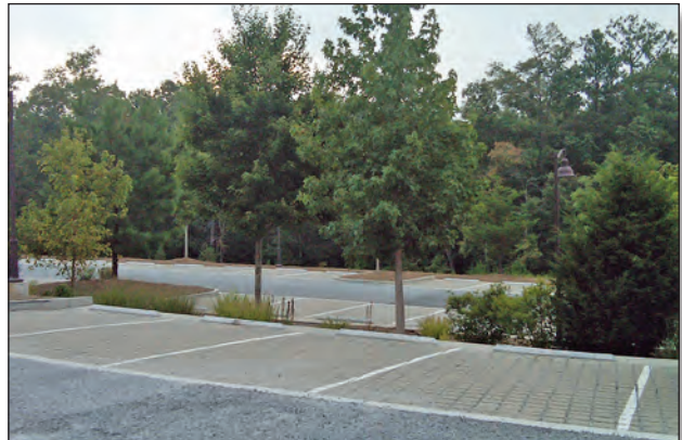
This parking lot, located in Gwinnett County, Georgia, uses permeable pavements and incorporates bioretention into a vegetated island.
