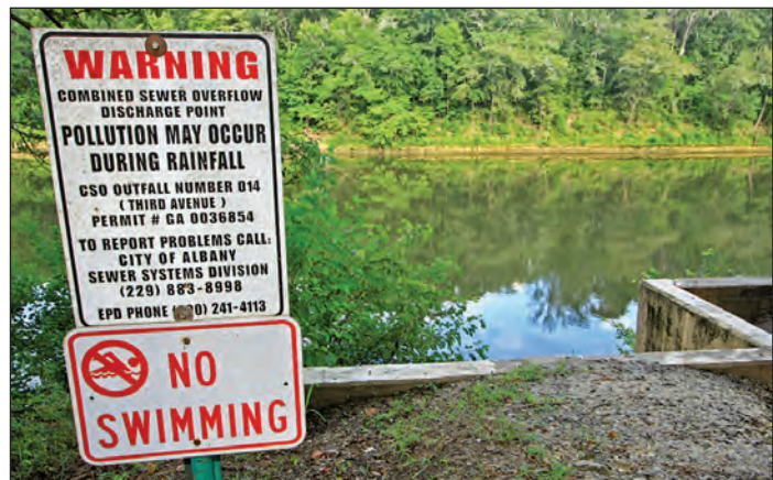
Figure 26. Overflows from combined sewer systems include a mix of stormwater runoff and untreated wastewater and are released into nearby waters when the flows exceed the capacity of the treatment plant. Warnings signs are posted near this combined sewer discharge point along the Flint River in Georgia due to the public health risks of contact with contaminated water.
