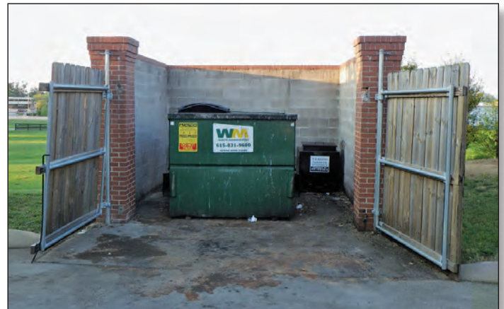
Business owners can prevent pollution by locating dumpsters away from storm drain inlets and making sure they are properly covered and maintained so they do not become a source of trash and other pollutants to local streams. Photograph from U.S. Geological Survey.
