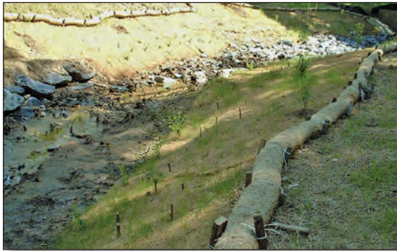
In this Howard County, Maryland, stream, coir fiber logs made of tightly bound coconut fiber provide short-term protection along the toe of the streambank until the newly planted live stakes take root and stabilize the streambank.
