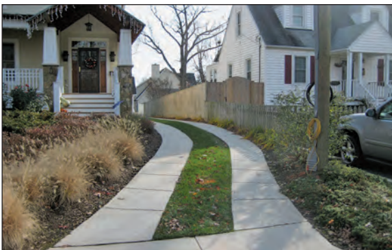
Another way to reduce impervious cover is by limiting pavement on driveways to only what is needed, as shown on this driveway in Arlington, Virginia.
