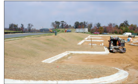
Hay is applied to temporarily stabilize soils on exposed sites and prevent erosion.
