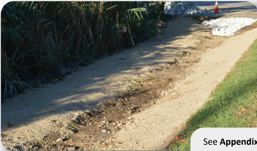
Figure 10: Newly graded ditch ready for seed application Image courtesy of Leslie Cario
