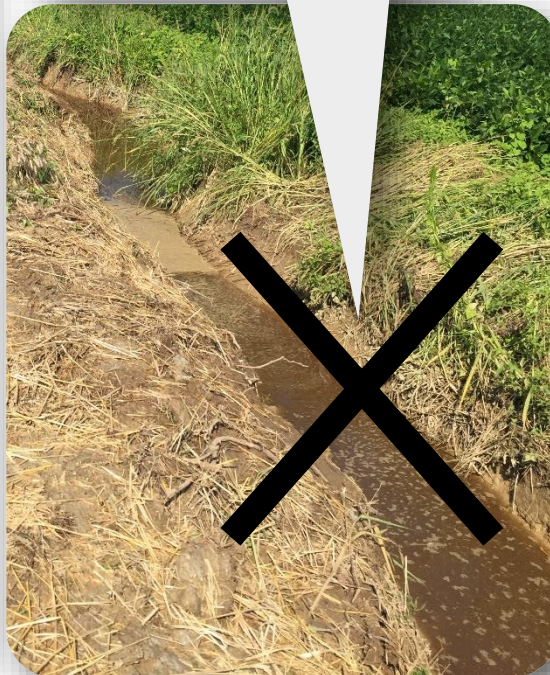
Bare side slopes and sediment-heavy runoff
