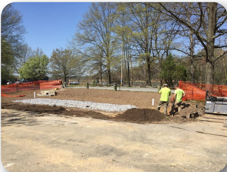
Figure 56 Roadside Ditch Undergoing Reconstruction
