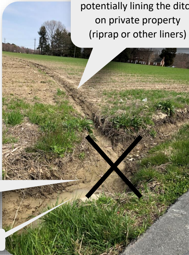
Figure 49: Scour at Agricultural Side Inlet
