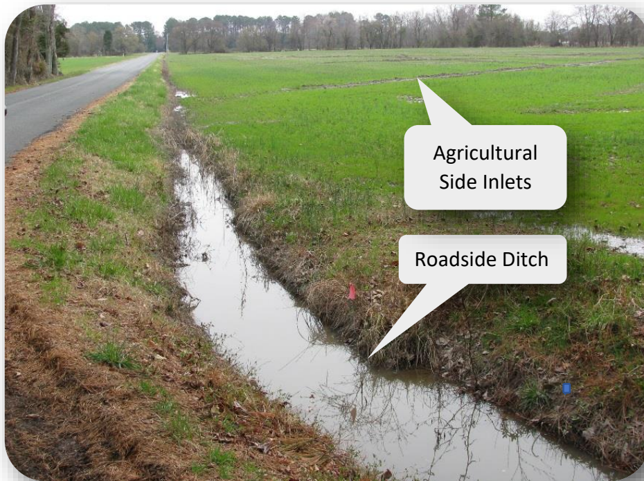
Figure 48 Agricultural Side Inlet Emptying into Roadside Ditch
