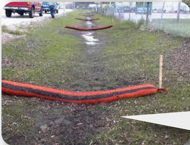
Figure 46 Compost Filter Sock Installation Image credit: https://archive.epa.gov
