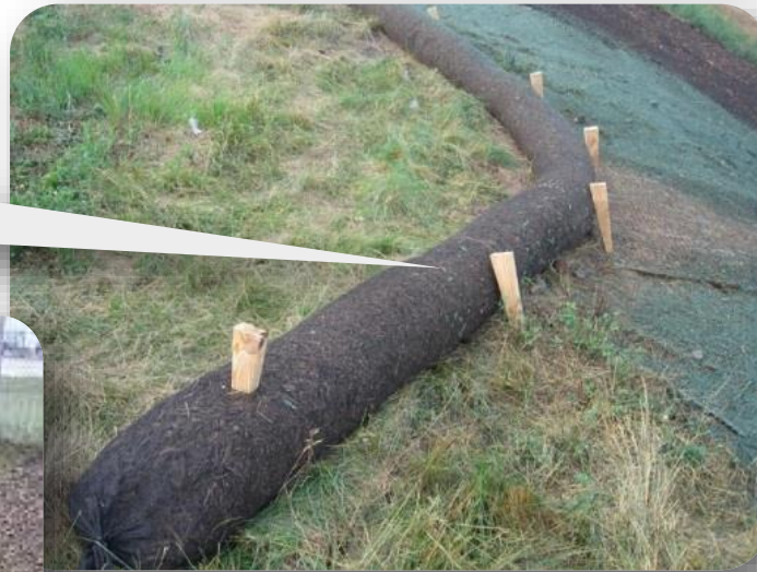
Figure 45 Compost Filter Sock Installation Image credit: Horsley Witten Group, CWP, NOAA
