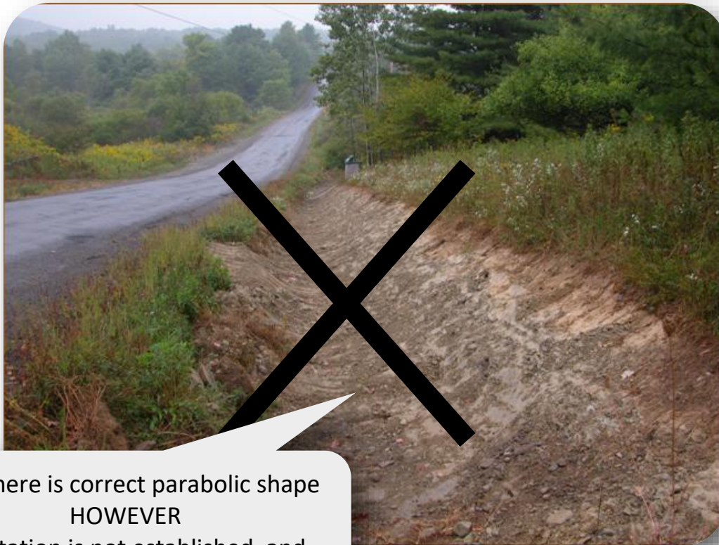
Figure 42 Ditch without Vegetative Stabilization Image credit: Environmental Inquiry Cornell University
