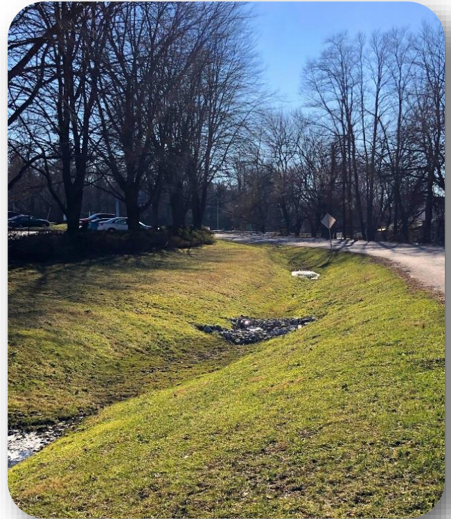
Figure 55: Reconstructed Roadside Ditch
