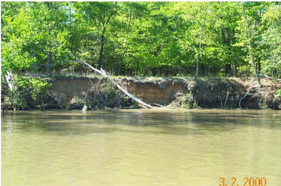
Figure 3-5. Shoreline erosion along Wright’s Island
