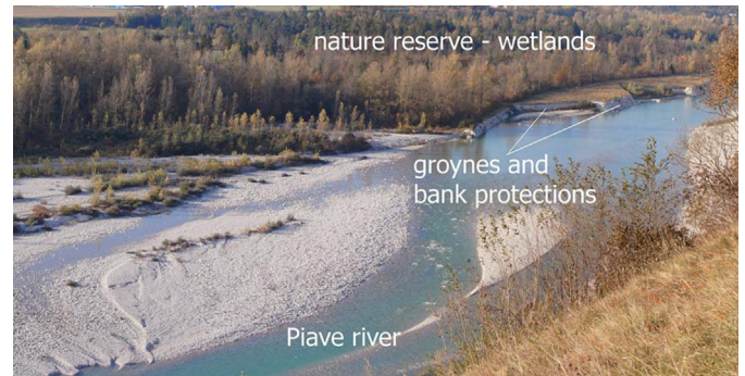
Fig. 7. Partial view of the portion of Piave river bordering the Nature reserve; in the upper part it is possible to see a portion of the impressive system of groynes and bank protections built to protect the reserve. The wetlands, not visible, are located inside the riparian forest.
