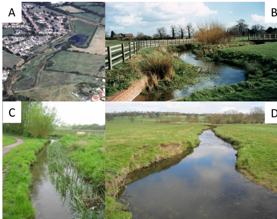
Fig. 4. (A) Aerial view of the Bear Brook and flood storage/overspill area. (B) Four years after the scheme and vegetation is shaping the low flow channel, establishing in the deposited silty margins. (C) In 2006 narrowing as a result of silt deposition and marginal plant growth. The open channel section has a clean bed. (D) The river at Coleshill 10 years after restoration showing little development from its dug dimensions; no deposition occurs due to the 'accurate' sizing of the channel for its flow regime and hence no marginal vegetation.
