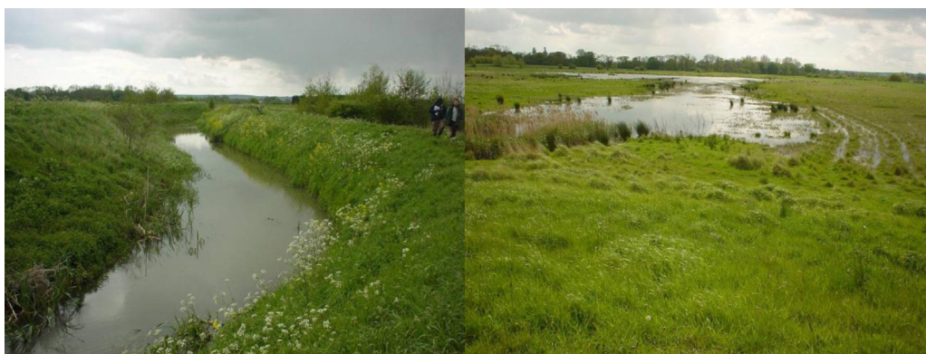
Fig. 9. Left an example of the large levees on the Long Eau prevent connection to the surrounding floodplain. On the right after restoration.
