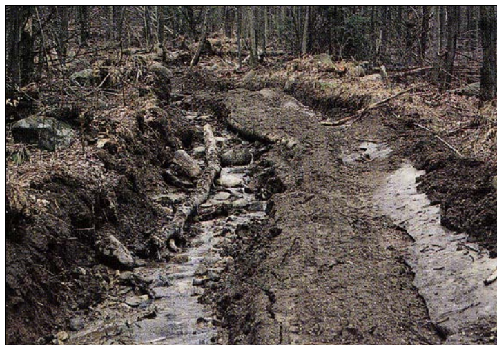
Figure 28. Forest Skid Trail Rutting Damage.
