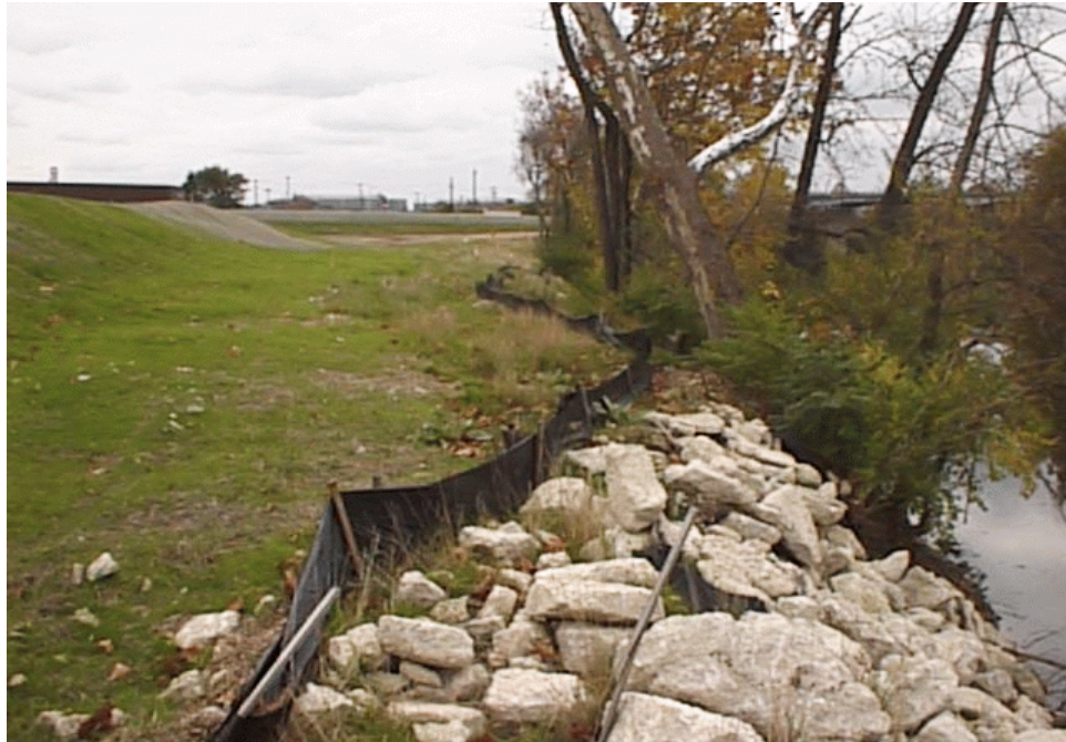
Temp. Grass, Silt Fence and Rock Channel Protection Combination
