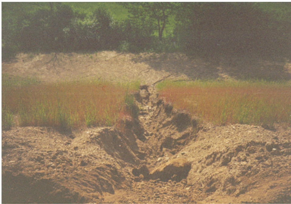
Gullies are formed by not using slope drains.
