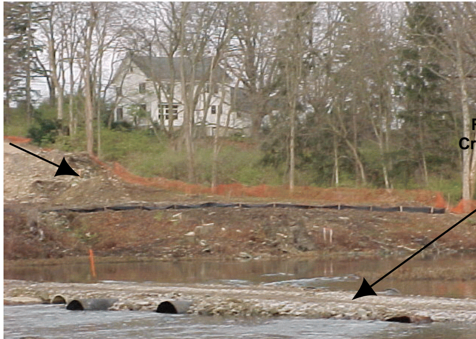
Sheet Flow and River Crossing(Not enough Pipe)
