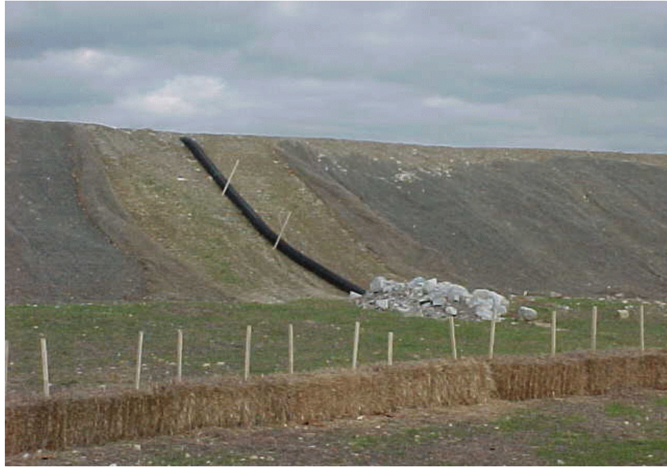
A good example of a slope drain.
