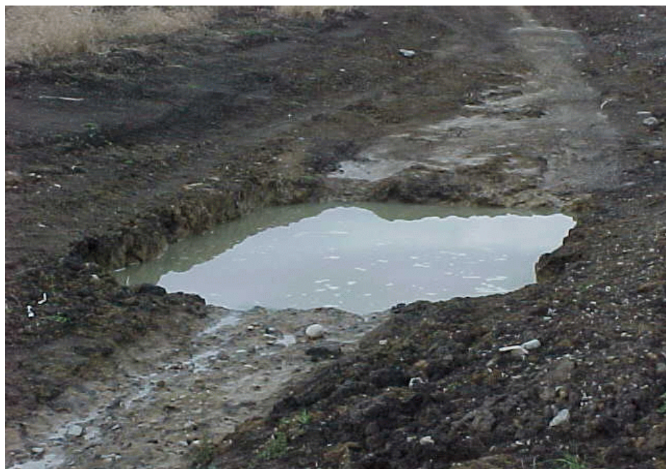
Poor example of a basin. Incorrect dimensions and no rock.
