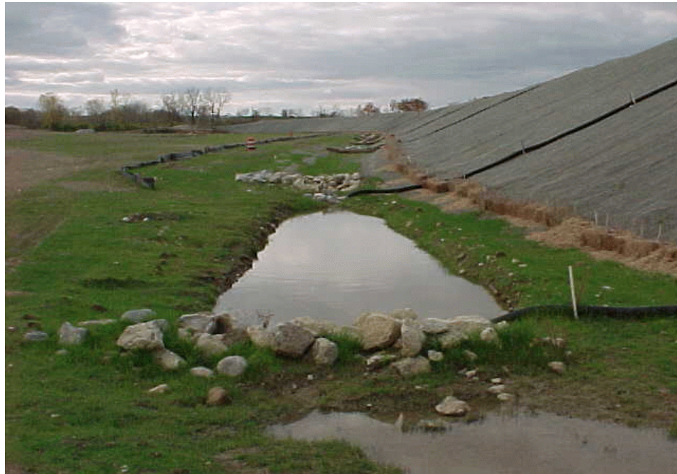
Good example of a basin. Right dimensions and rock type.
