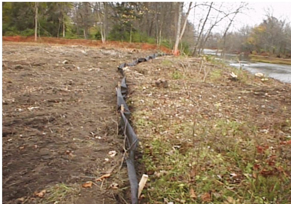
Perimeter Silt Fence Protecting the River Good Location but Bad Construction
