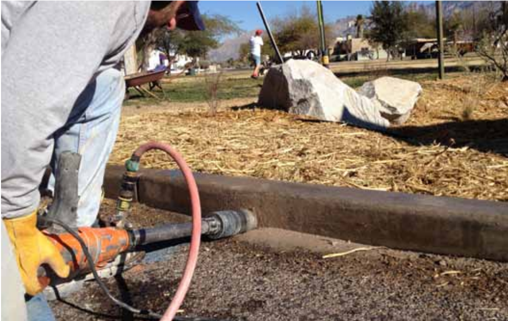
Drilling a 4" core at a slight downward angle to enhance water flow into basin.
