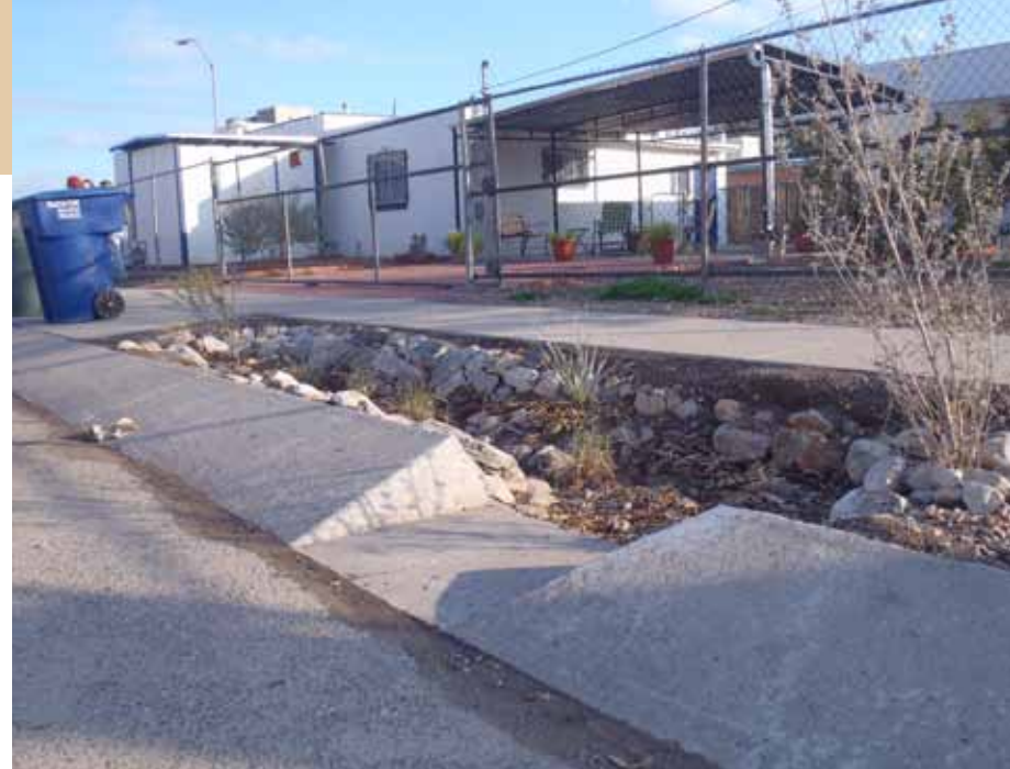
Curb cuts can still work on wedge curbs.
