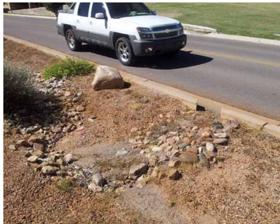
Simple, angled curb cut enhances capture of stormwater moving along the gutter.
