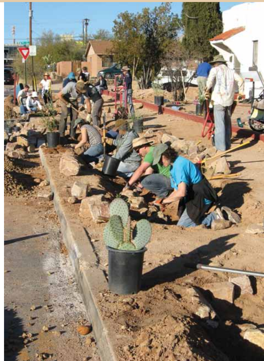
Volunteers install bioretention basins in the right-of-way at a workshop in Tucson led by Watershed Management Group.
