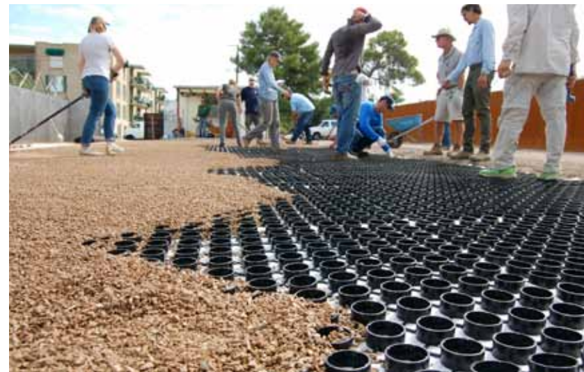
Participants in a professional green infrastructure training learn how to install a permeable parking surface. A recycled plastic base retains a gravel surface that promotes infiltration.
