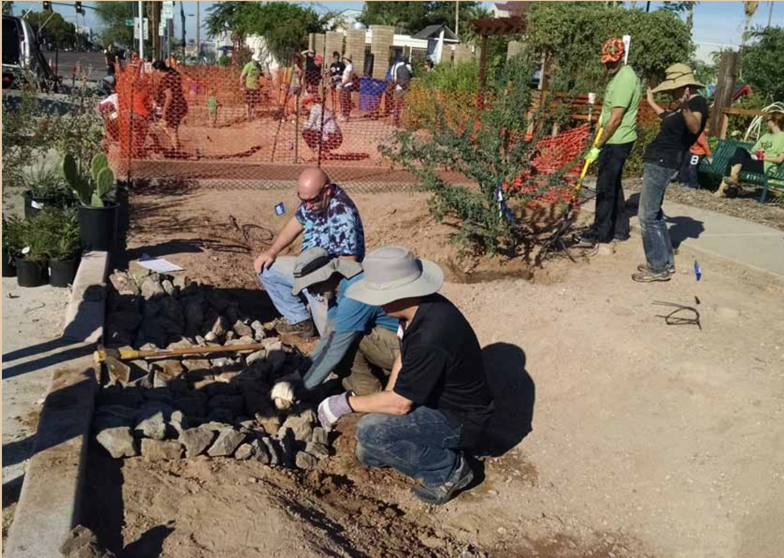
This 400 sq ft rain garden has the potential to harvest 4,500 gallons of stormwater each time it rains. The project was installed by WMG in partnership with the City of Mesa, in front of the Mesa Urban Gardens.
