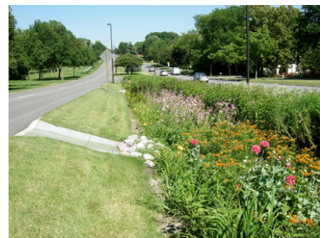
Bioswales and bioretention gardens help manage stormwater on site, rather than collecting it in pipes and sending it all downstream at once. Photo courtesy of Flickr/Aaron Volkening.
