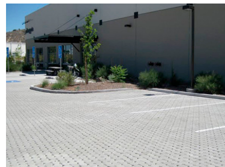
Parking lot with concrete pavers allowing stormwater to infiltrate. Note the curb cut to the right of the tree, allowing excess stormwater to flow into a bioswale. Photo courtesy of the University of Nevada Extension.
