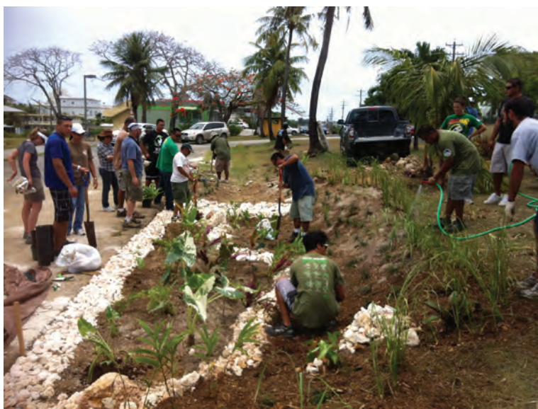
Figure 2. Island agencies, NOAA, HW, and the Center construct Saipan's first rain garden.
