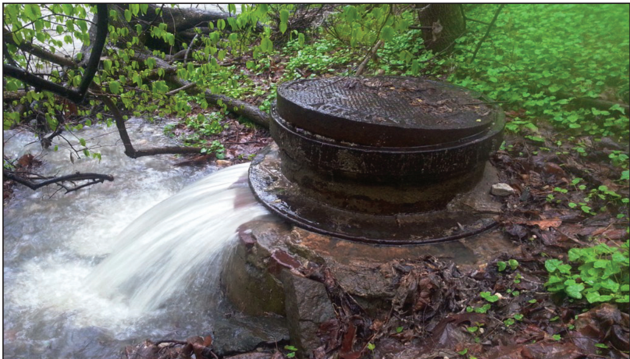
Sewer overflow in Baltimore (Photo source: Blue Water Baltimore)
