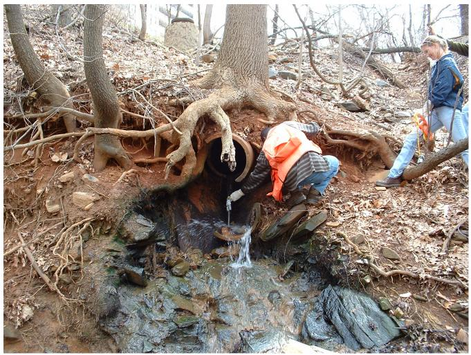
Figure 3. Illicit discharge detection in the City of Baltimore.
