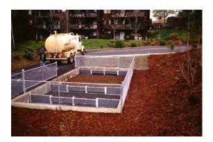
**Description**: Design variant of the surface sand filter using organic materials in the filter media.
