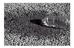
**Description**: Pervious concrete is a mixture of coarse aggregate, Portland cement and water that allows for rapid infiltration of water and overlays a stone aggregate reservoir. This reservoir provides temporary storage as runoff infiltrates into underlying permeable soils and/or out through an underdrain system.
