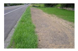
**Description:** Specialized media filtration BMP typically used in longitudinal applications to treat stormwater along an impervious area (road, parking lot, etc.).
