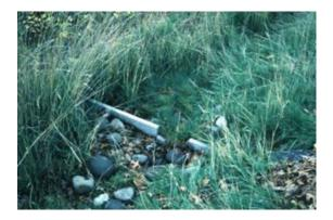
**Description**: Vegetated open channels that are explicitly designed and constructed to capture and treat stormwater runoff within dry or wet cells formed by check dams or other means.
