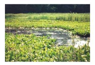
**Description:** Constructed wetland systems used for stormwater management. Runoff volume is both stored and treated in the wetland facility which consists of a shallow impoundment with a permanent pool designed to mimic natural wetlands.
