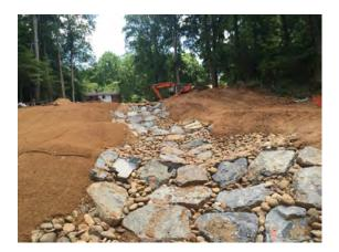
**Description**: Regenerative stormwater conveyance (RSC) provides treatment, infiltration and conveyance through the combination of sand, wood chips, native vegetation, riffles (with either cobble rocks or boulders), and shallow pools. RSCs are designed to convey water while minimizing the effects of erosion.
