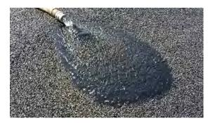
**Description**: Porous asphalt is asphalt with reduced sands or fines and larger void spaces, which allow water to drain through it. Porous asphalt allows water to infiltrate into the subsoil below through the paved surface and base layer. This aggregate base layer acts as a structural layer and container to temporarily hold stormwater.
