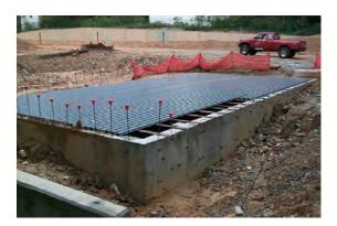
**Description**: Detention storage located in underground tanks or vaults designed to provide water quantity control through detention and/or extended detention of stormwater runoff.
