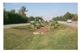
properly. The picture to the right shows an example of the main treatment area of a dry enhanced swale. Main treatment areas treat stormwater runoff through different methods including vegetated conveyance, infiltration, filtration, and settling. For example, the main treatment area of a pond treats stormwater runoff primarily through settling, and the main treatment area of a sand filter treats runoff through filtration. Specific maintenance concerns within a treatment area are
