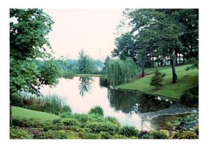
**Description:** Constructed stormwater retention basins that have a permanent pool (or micropool). Runoff from each rain event is detained and treated in the pool primarily through settling and biological uptake mechanisms.
