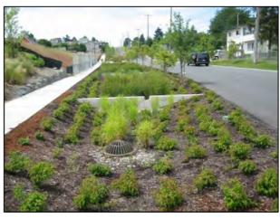
bottom of the swale. Because they are dry most of the time, they are often the preferred option in residential settings. The second type of enhanced swale is a wet swale. Wet swales are designed to retain water or marshy conditions that support wetland vegetation. Because this practice is meant to retain water, they are generally used in areas with a high water table or poorly drained soils. Wet swales achieve pollutant removal both from sediment accumulation and biological removal.
