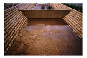
**Description**: Multi-chamber structure designed to treat stormwater runoff through filtration, using a sediment forebay, a sand bed as its primary filter media and, typically, an underdrain collection system.
