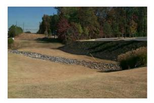
**Description**: A surface storage basin or facility designed to provide water quality treatment and water quantity control through detention of stormwater runoff. Dry detention basins differ from dry extended detention (ED) basins (Section 4.6) in that they do not provide 24-hour detention of the channel protection volume (CP.).
