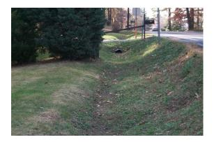
**Description**: Grass channels designed to enhance water quality through the settling of suspended solids.
