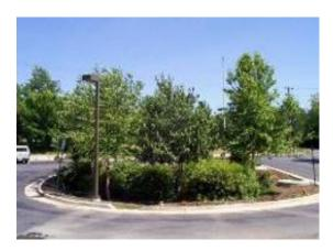
**Description**: Shallow stormwater basin or landscaped area that utilizes engineered soils or native, well-draining soil and vegetation to capture and treat runoff.
