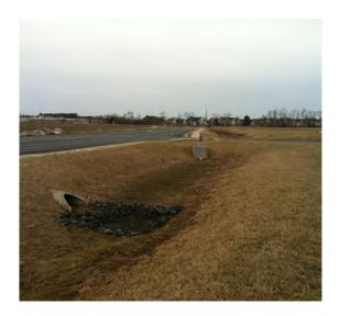
**Description**: A surface storage basin or facility designed to provide water quality treatment and water quantity control through extended detention (ED) of stormwater runoff. Dry ED basins differ from dry detention basins in that they provide 24-hour detention of the channel protection volume (CP).
