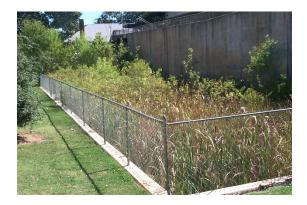
**Description:** One or more cells filled with crushed rock designed to support wetland plants. Stormwater flows subsurface through the root zone of the constructed wetland, where pollutant removal takes place.
