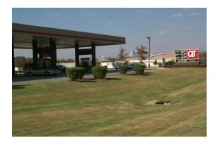
**Description**: Vegetated filter strips are uniformly graded and densely vegetated sections of land, engineered and designed to treat runoff from and remove pollutants through vegetative filtering and infiltration.
