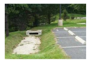
**Description:** Infiltration practices, which may also be classified as a runoff reducing low impact development practices, are shallow excavations, typically filled with stone or an engineered soil mix, that are designed to intercept and temporarily store post-construction stormwater runoff until it infiltrates into the underlying and surrounding soils. If properly designed, they can provide significant reductions in post-construction stormwater runoff rates, volumes and pollutant loads.
