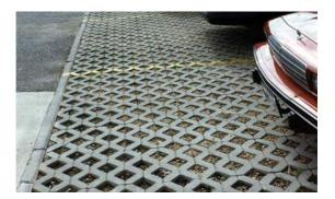
**Description**: A pavement surface composed of structural units with void areas that are filled with pervious materials such as gravel, sand, or grass turf. Permeable paver systems are installed over a gravel base course that provides structural support and stores stormwater runoff that infiltrates through the system into underlying permeable soils
