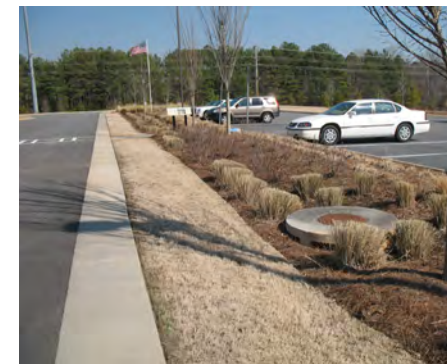
Figure 3.3-27 Parking lot bioretention in Johns Creek, GA.
