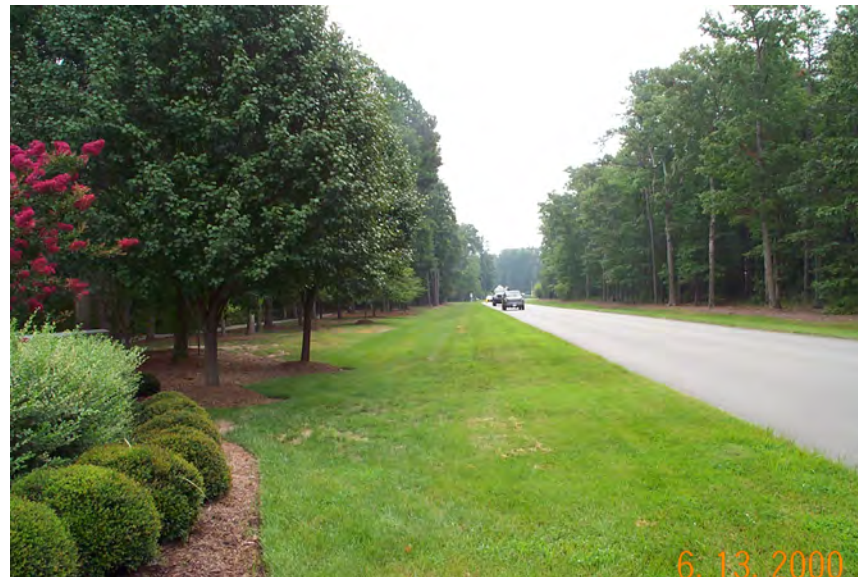
Figure 3.3-25 Road with grass swales instead of curb-and-gutter
