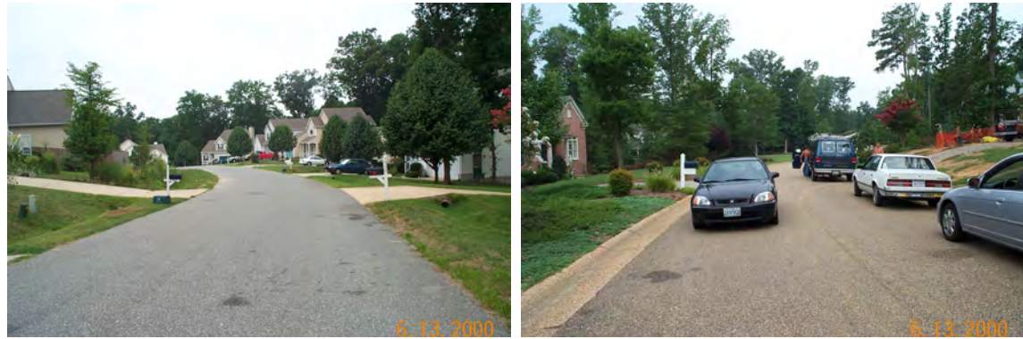
Figure 3.3-17 Narrow streets reduce impervious cover area.
