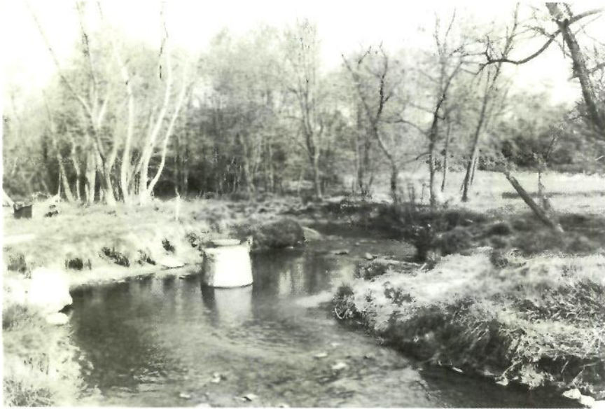
FIGURE 11A. View downstream in 1961 showing manhole far to the left of the channel. By 1994, in figure 11B, the channel had moved so far that the manhole stood in the center of the stream.
