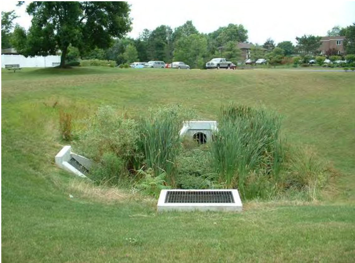
Figure 8. A short internal flowpath from inlet to outlet decreases wetland pollutant removal performance
