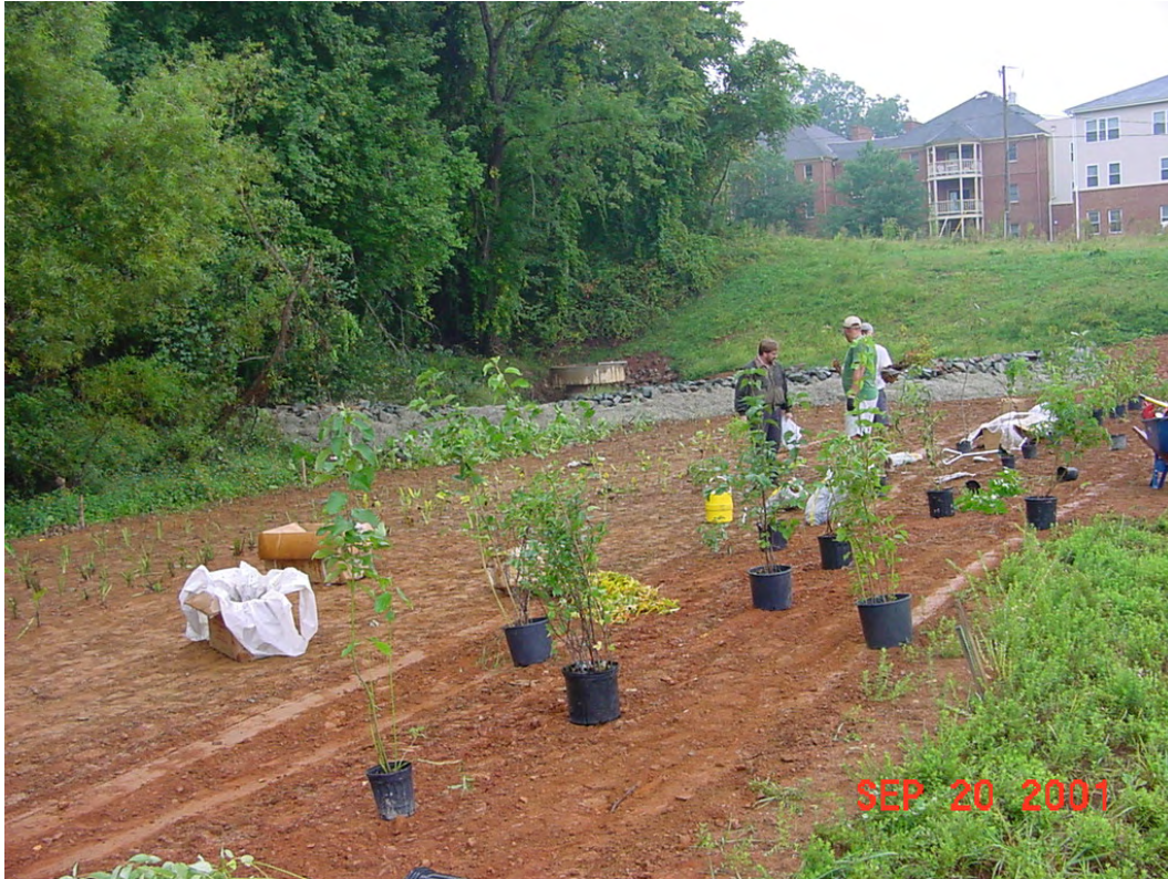
Figure 6. Retrofitting a dry pond into a wetland
