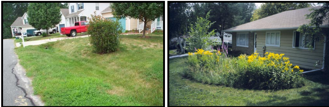
Figure 12. Roadside swales (left), and rain gardens (right) are used to infiltrate runoff (Rain garden photo source: Roger Bannerman)
