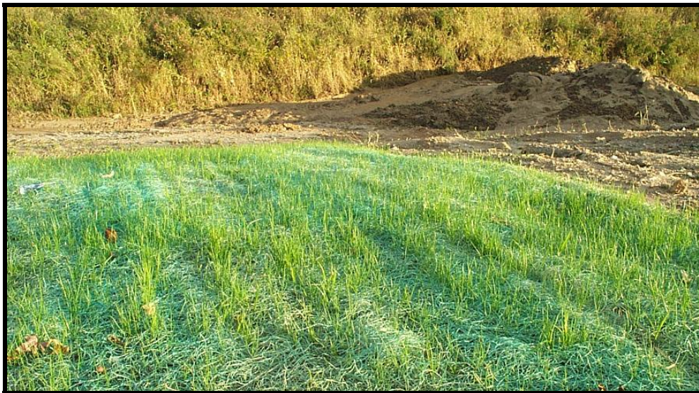
Figure 14. Exposed slope stabilized with erosion control matting
