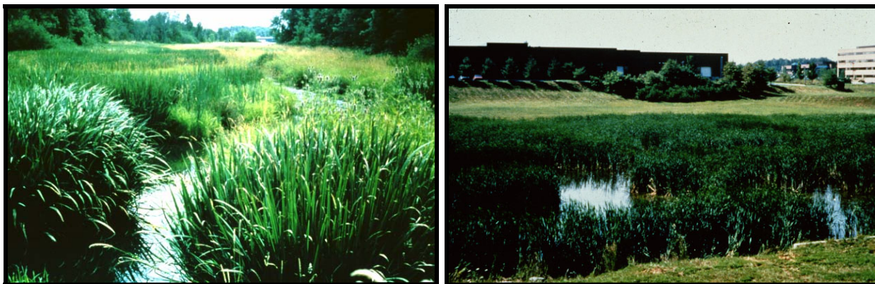
Figure 23. Comparison of a well designed (left) and a poorly designed (right) storm water wetland
