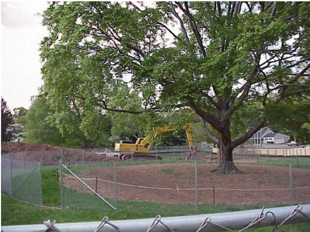
Figure 15. Fencing surrounds a mature tree that is to be preserved.
