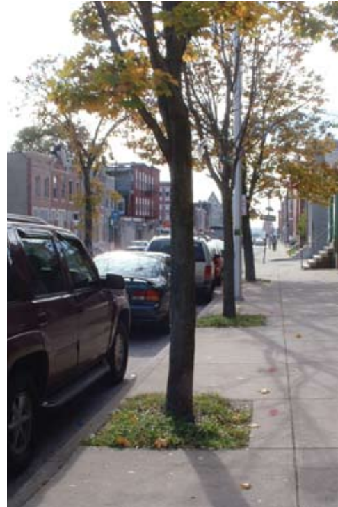
Figure 5. A typical urban tree pit is about 4 feet by 4 feet and does not provide adequate soil volume for most trees.
