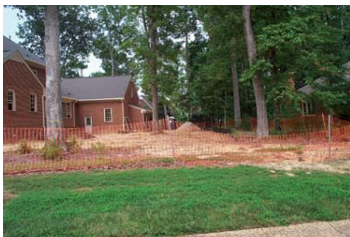
Figure 14. Orange plastic mesh fencing delineates tree protection areas.
