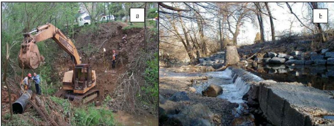
Figure 29: Structural Repair and Fish Barrier Removal at Utilities
