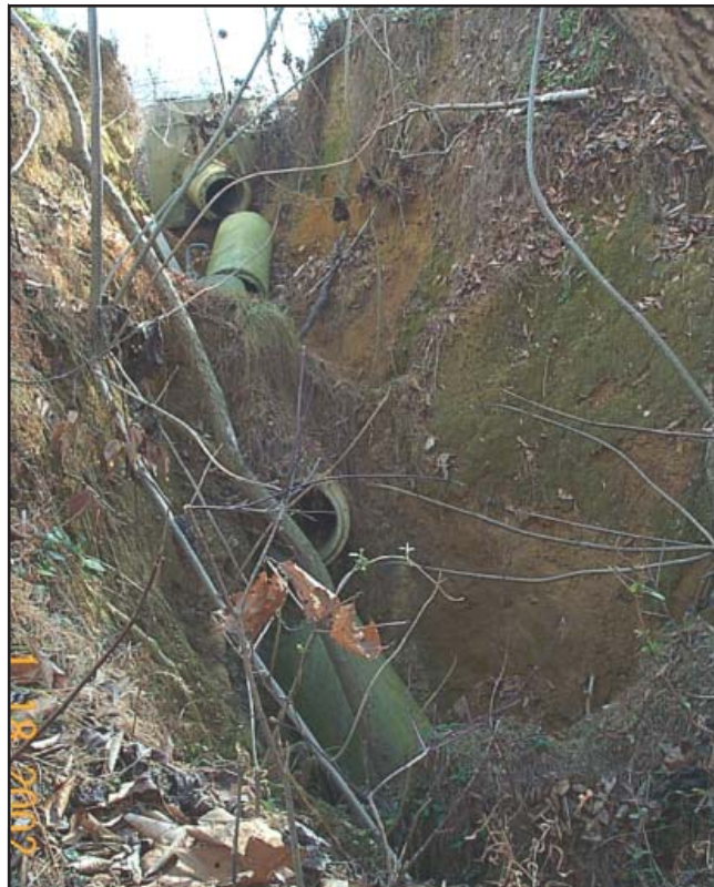
Figure 16: Local Stream or Outfall Repair
