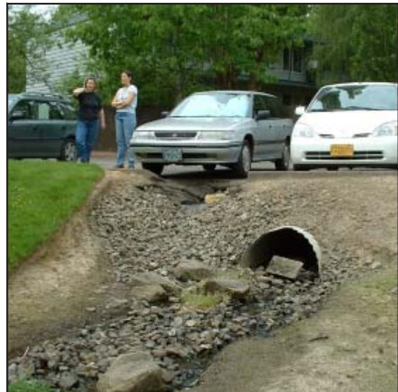
Figure 35: Minor Culvert Repair
