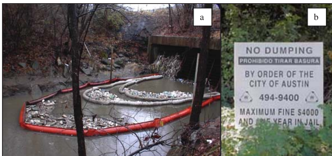
Figure 33: Deploying a Trash Boom
