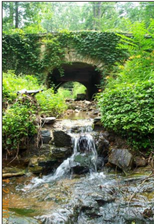
Figure 37: Grade Control and Potential Fish Barrier
