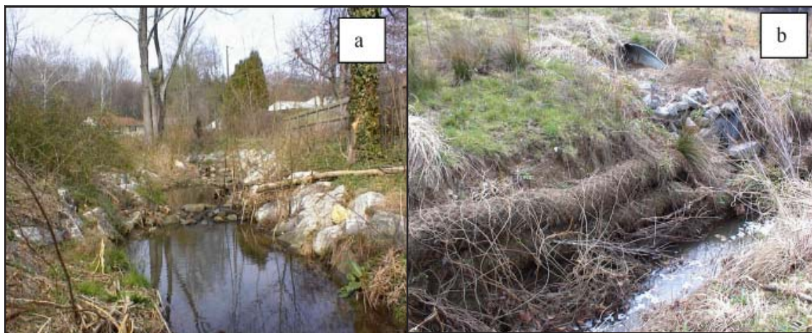
Figure 21: Example Hard and Soft Bank Stabilization Practices
