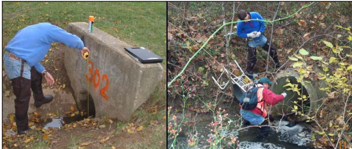
Figure 14: Detailed Discharge Investigations
