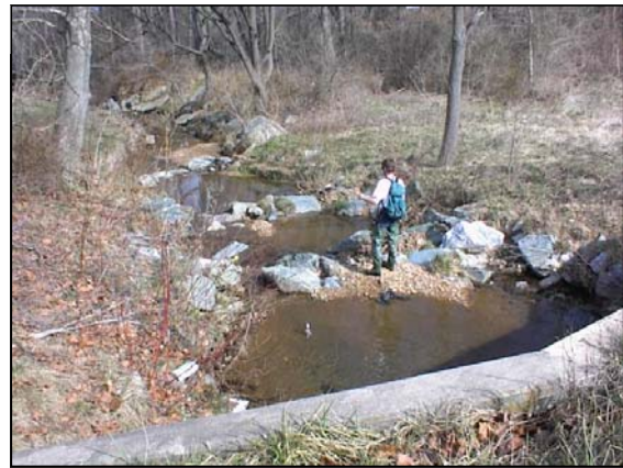
Figure 22: Example Grade Control Practice Steps pools can be used as grade control.
