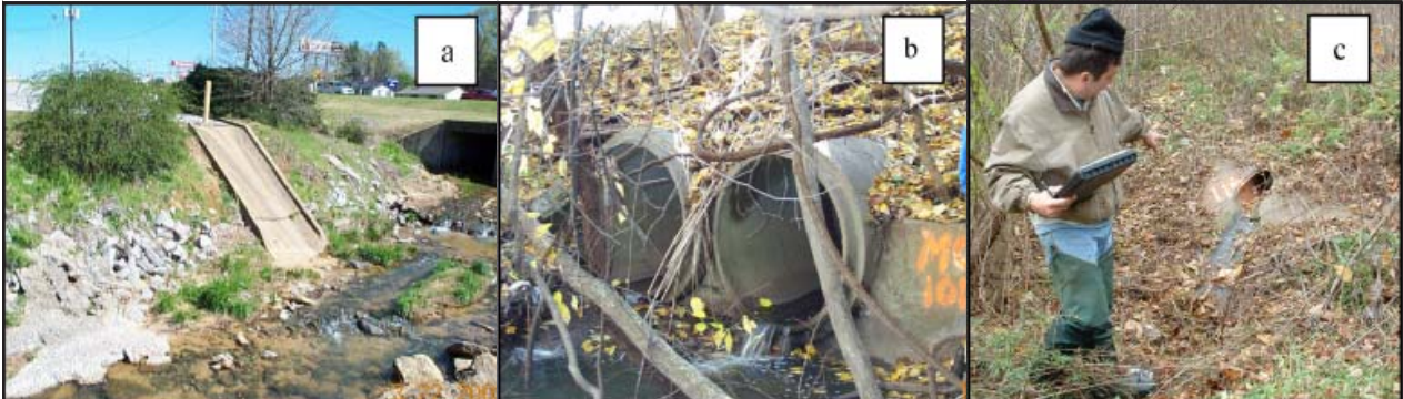
Figure 13. Types of Outfalls to Expect Storm water outfalls come in a variety of shapes and sizes. For example, not all outfalls will be closed pipes, such as the open channel draining the corner of a commercial parking lot (Panel A). Some outfalls may be single or double concrete pipes draining directly to the stream (Panel B), while others may be quite small, such as the six-inch diameter pipes discharging into the buffer in Panel C.
