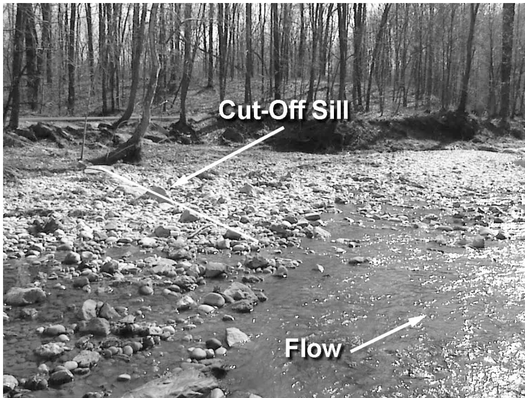
Photo 4.27: Cut-off sill within new lateral bar.
