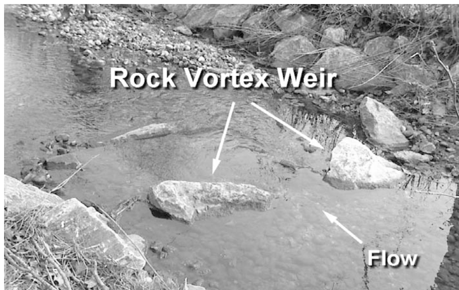
Photo 4.13: Properly designed and installed rock vortex weir.
