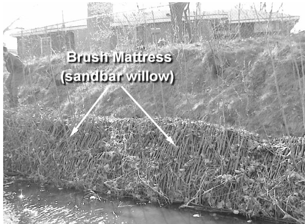
Photo 4.33: Brush mattress installation using sandbar willow cuttings.
