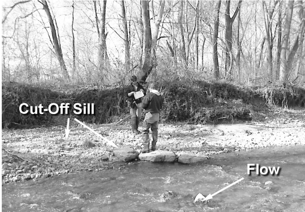
Photo 4.26: Cut-off sill installation that has caused sediment deposition along channel margin.
