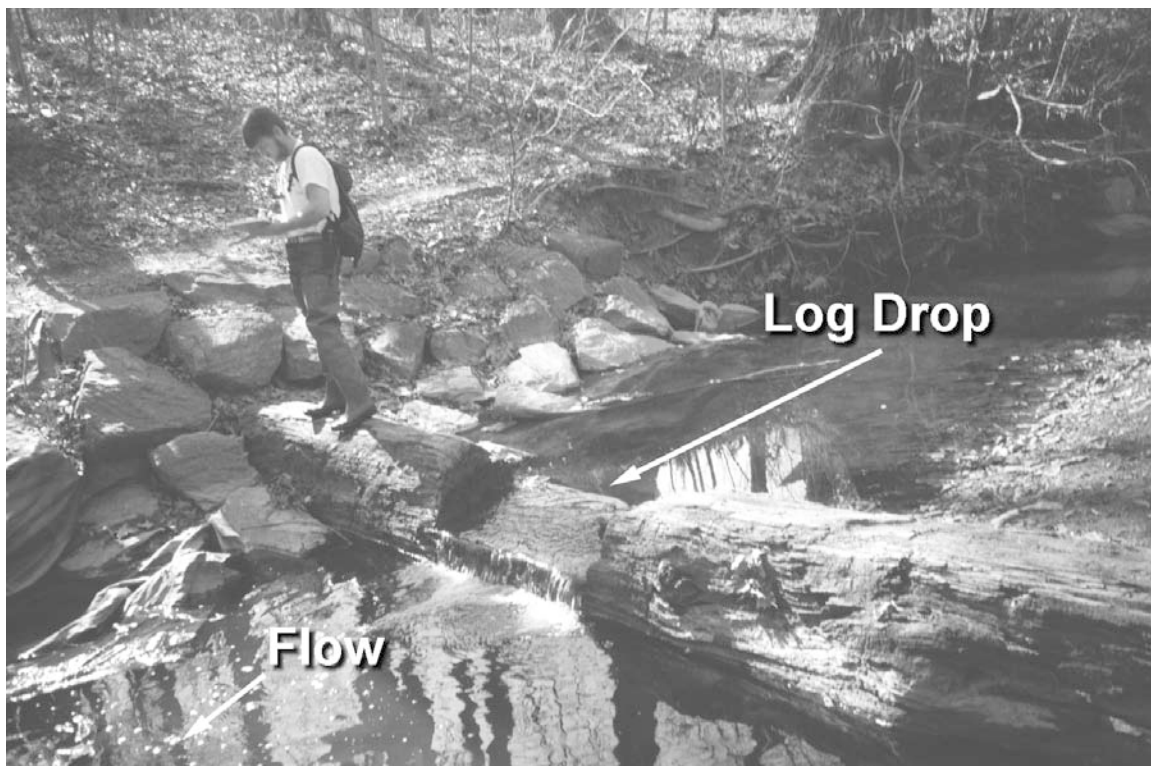
Photo 4.20: Log drop structure.
