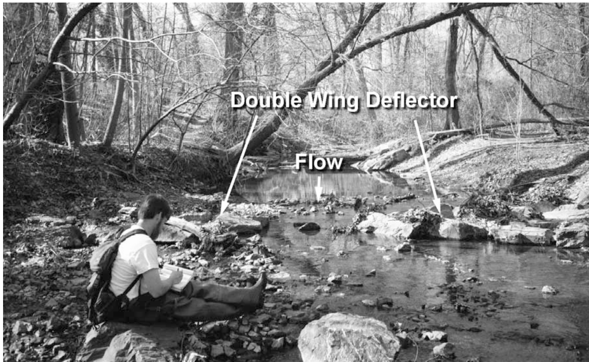
Photo 5.11: Double wing deflector constructed low in profile. Note lack of pool formation downstream of structure.
