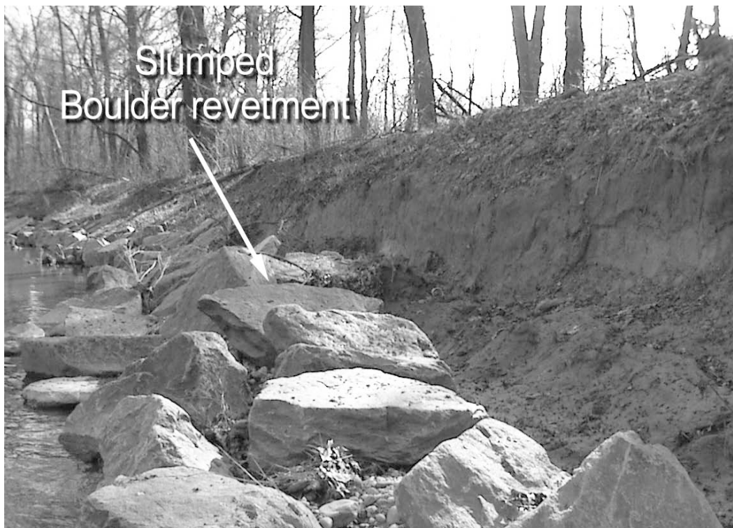
Photo 4.7: Large boulder revetment that has slumped due to scouring at the streambank toe and saturated soil conditions within the streambank. Revetment moved in mass.
