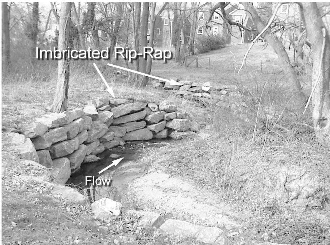
Photo 4.4: Well designed and installed imbricated rip-rap revetment.
