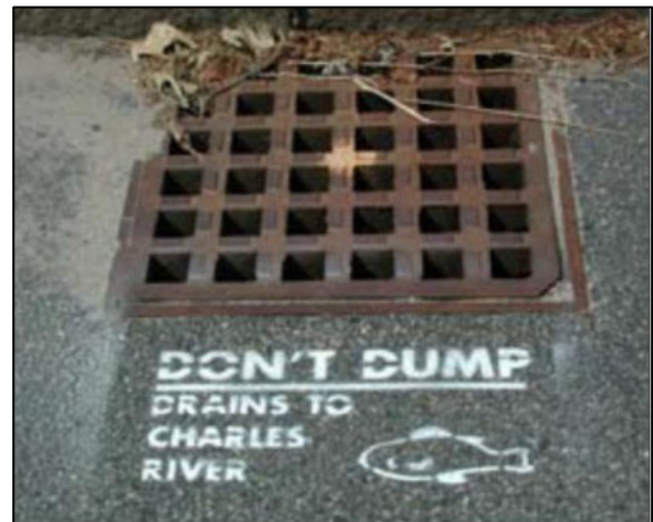
Figure 1: Storm Drain Marking
