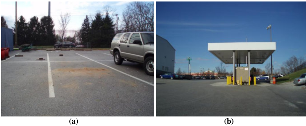
Figure 3.18. (a) Sediment on parking lot at the County's Ridge Rd. facility; and (b) Covered fueling area at the County's Ridge Rd. facility - Use a perimeter drain or slope the pavement inward so that runoff drains to a blind sump. It might be necessary to install and maintain an oil control device in catch basins that might receive runoff from the fueling area.
