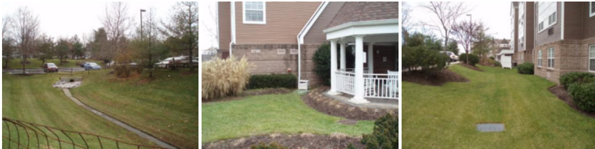
Figure 3.12. (a) Concrete channel in stormwater pond could be retrofit to provide water quality treatment at NSA_21; and (b & c) Rain garden or bioretention potential at NSA_21.
