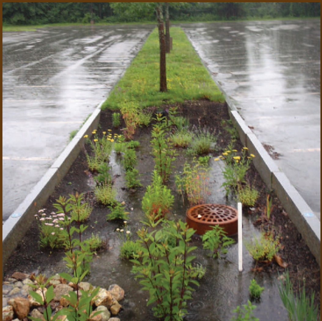
FIGURE 3-5 Completed Bioretention Retrofit Installation 2008
