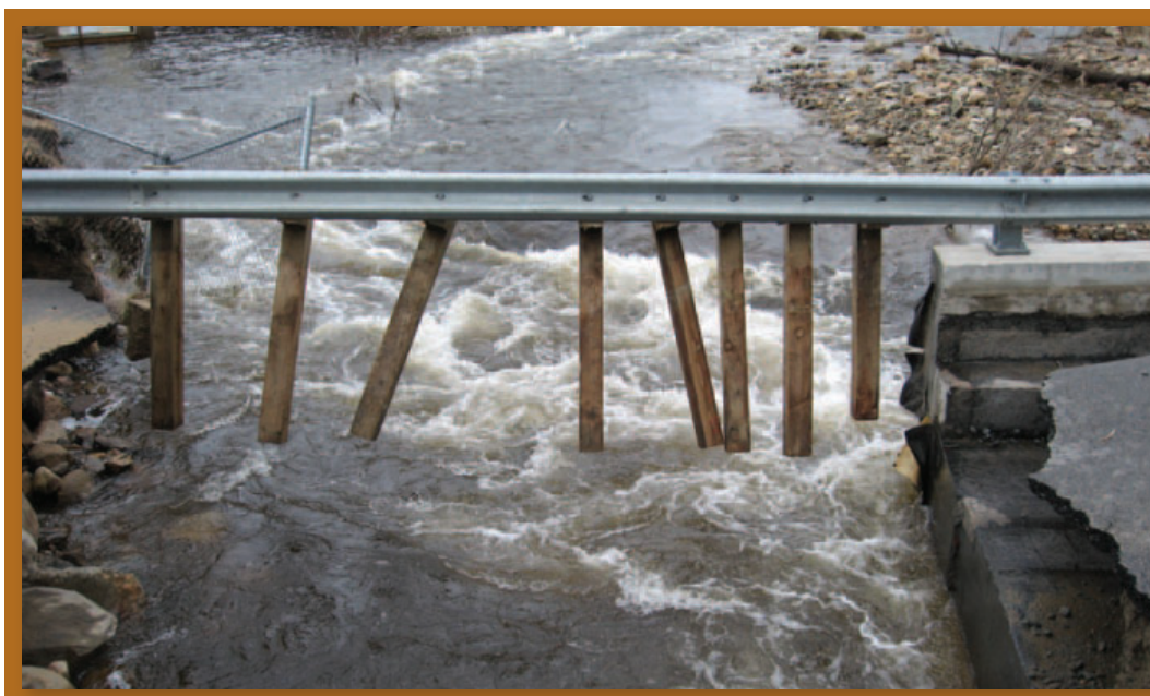
FIGURE 5-2 Mill Pond Road after dam failure at Nottingham Lake, Nottingham, NH, 4/18/2007. Hanging in the picture is the guard rail and support posts for the washed-out road.
