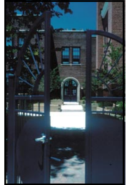
Barrister Court: Baltimore, MD
