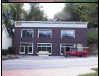
CWP Office Building: Ellicott City, MD
