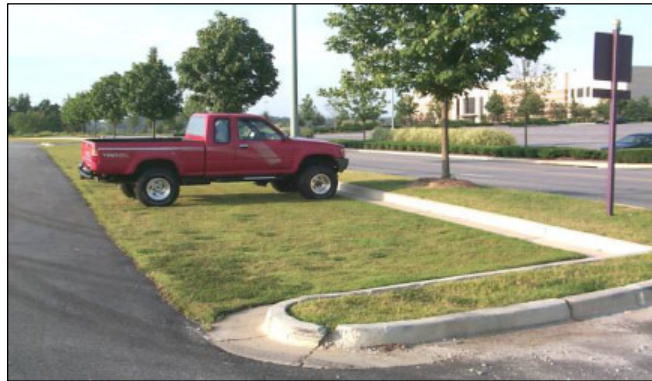
Figure 5. 30 Grass pavers for parking (Source: Georgia Stormwater Manual, 2001)
