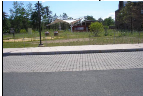
Figure 5. 59 Asphalt, Permeable Pavers, Porous Concrete, Albany, NY
