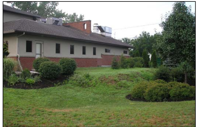
Figure 5. 39 Rooftop disconnection for storage and infiltration, Guilderland, NY, NYSDEC
