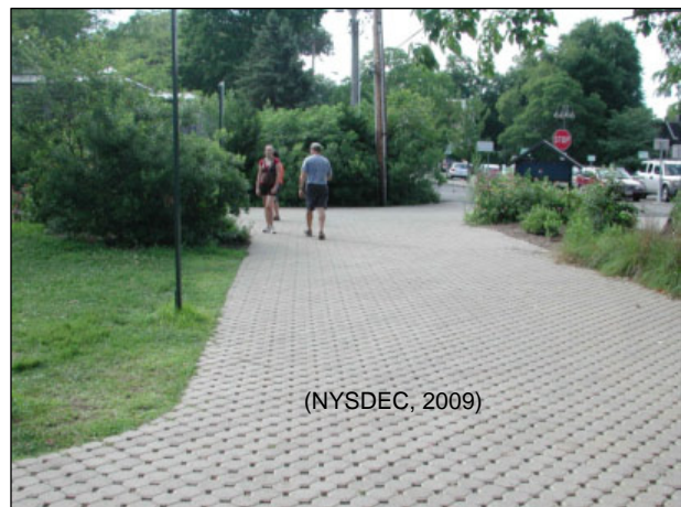
Figure 5. 60 Walkway with permeable pavers - Scenic Hudson Park, Cold Spring, NY
