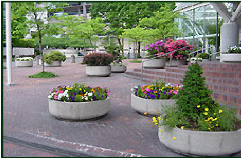
Figure 5. 54 Contained stormwater planters made of concrete
