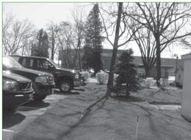
Parking lot runoff treated by a swale
