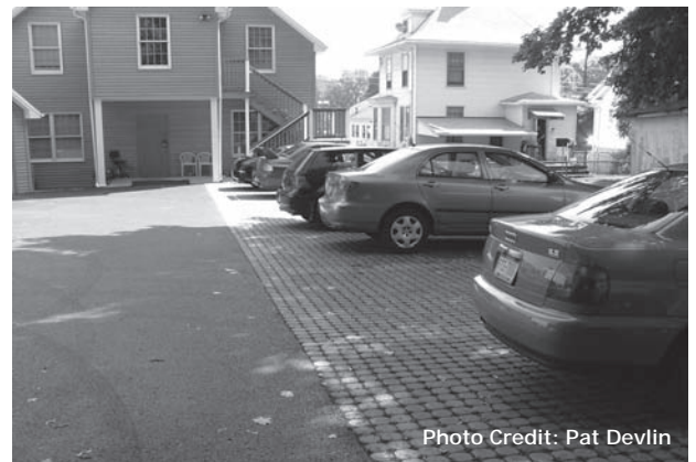
This office parking lot employs pervious pavers to infiltrate parking lot runoff.
