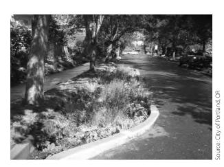
Street bumpouts both act as a traffic calming measure and provide stormwater treatment
