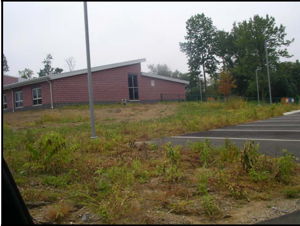
Figure 34. Space for stormwater treatment practice at the Londonderry School
