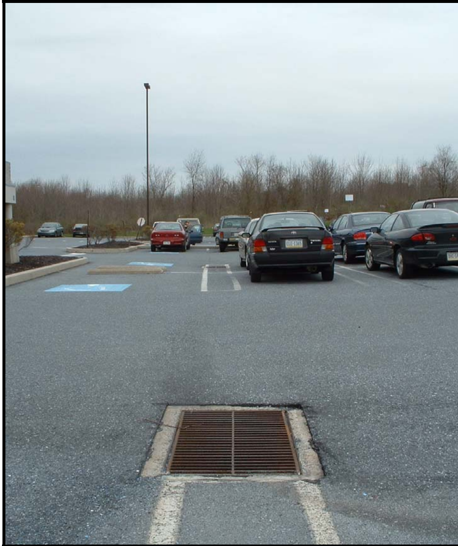
Figure E-5 - Large expanse of pavement drains untreated to the storm drain in Upper PCN
