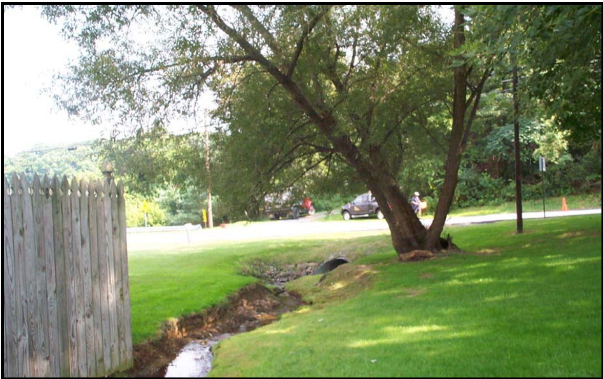
Figure 39. Small eroding stream located on the Glaser property
