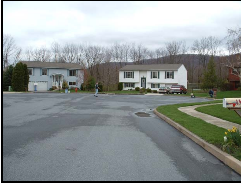
Figure 41. A 100-foot diameter cul-de-sac in Paxton Creek North (a lost opportunity for bioretention) illustrates the need for Better Site Design
