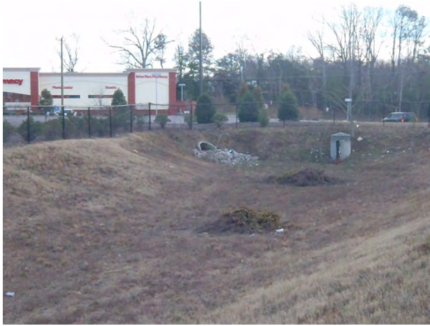
Figure 1: Shrub clippings in detention pond
