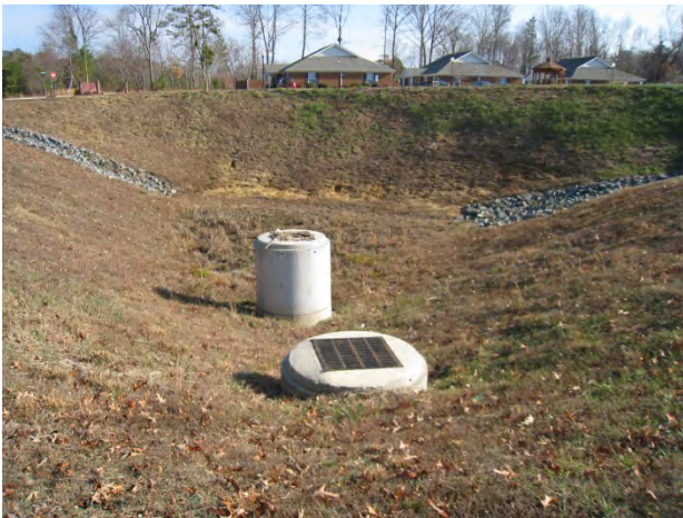
Figure 3. Detention basin in communal area
