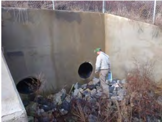
Figure 15: Concrete headwall above S-103
