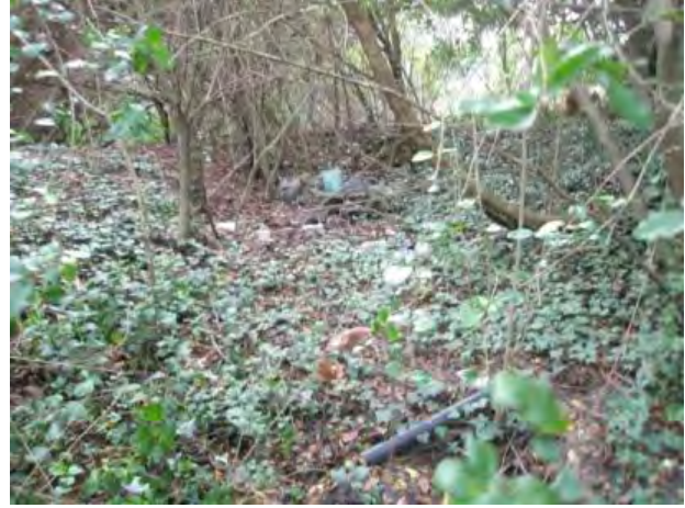
Figure 4: BMP ponding area and riser (blue pipe in background)
