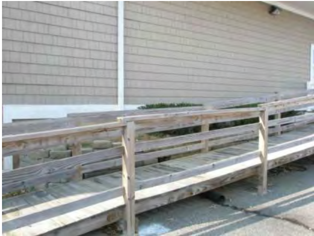
Figure 1: Left side of building downspout
