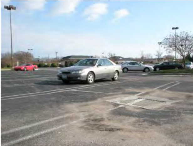
Figure 1: Typical parking lot inlet
