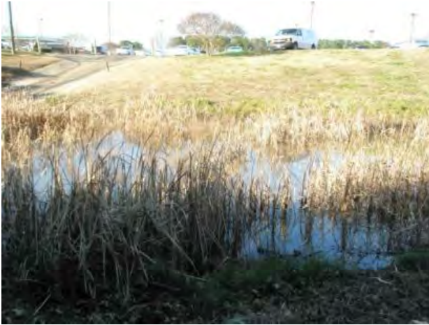
Figure 1: Existing stormwater basin
