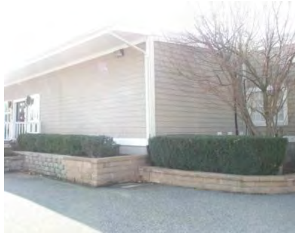
Figure 1: Right side downspout
