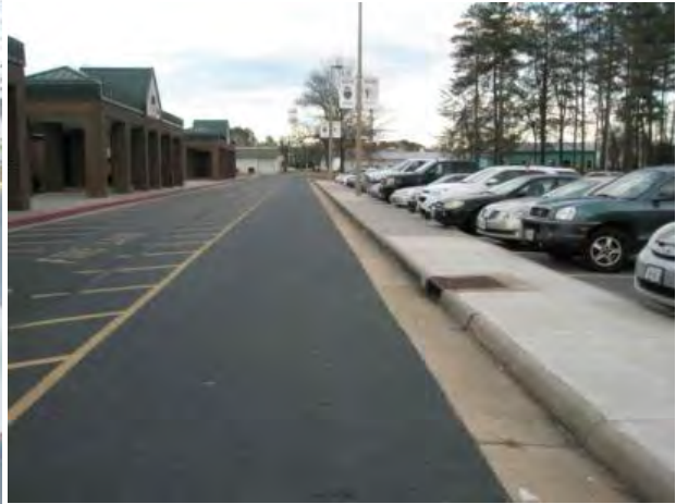
Photo 2: Driveway drainage to Biofilter B
