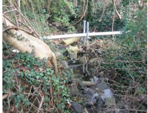
Figure 1: Downstream of existing BMP
