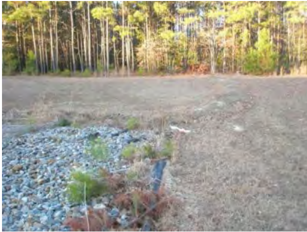
Figure 1: Infiltration trench w/ low earthen berm
