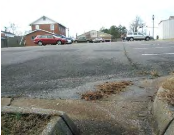
Figure 1: Existing drainage from parking lot
