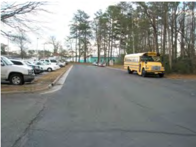
Photo 5: Location of Dry Swale (left) & drainage to Biofilter D.
