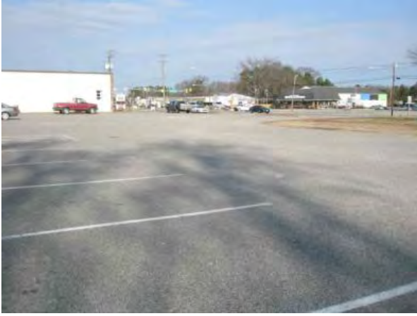
Figure 3: Paved area in front of building
