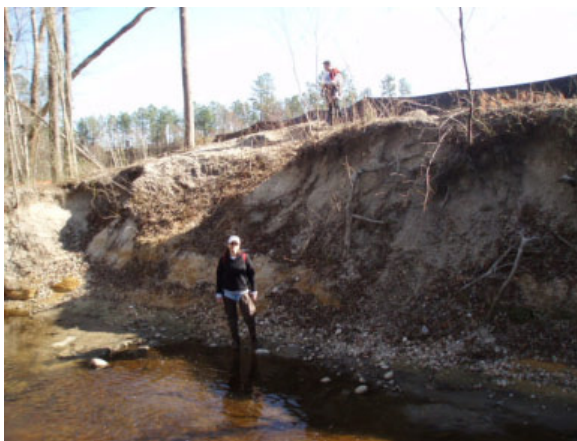
Project 25A: Potential RPA encroachment (OTC-2, MI-1)
