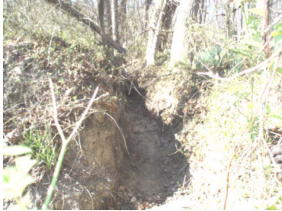
Project 13: Headcut channel from Rt. 95 runoff (OTC-2, ER-1)
