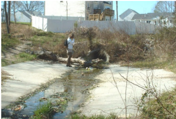
Project 24E: Reach BL-06, OT-1: Concrete pipe.
