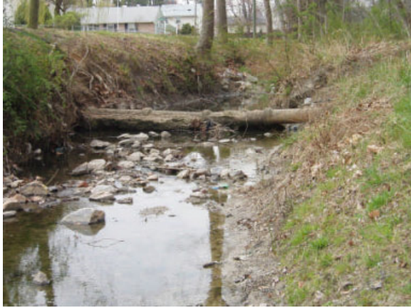
Project 27B: Reach TB-06, UT-02: The pipe has joint failure, cracks and a milky gray color and staining.
