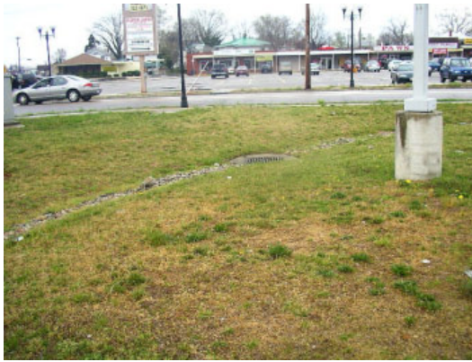
Project 28: Stormwater maintenance at CVS Swale
