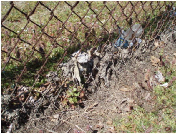
Project 22B: Sewage residue on fence near pump station
