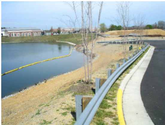
Project 17: Slope stabilization behind Best Buy
