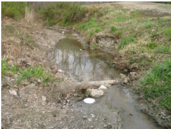
Project 27A: Reach TB-06, UT-01: Possible leaking sewer line near trapezoidal section of tributary.
