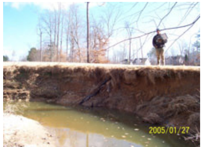
Figure 10. Little Lick Stream Erosion
