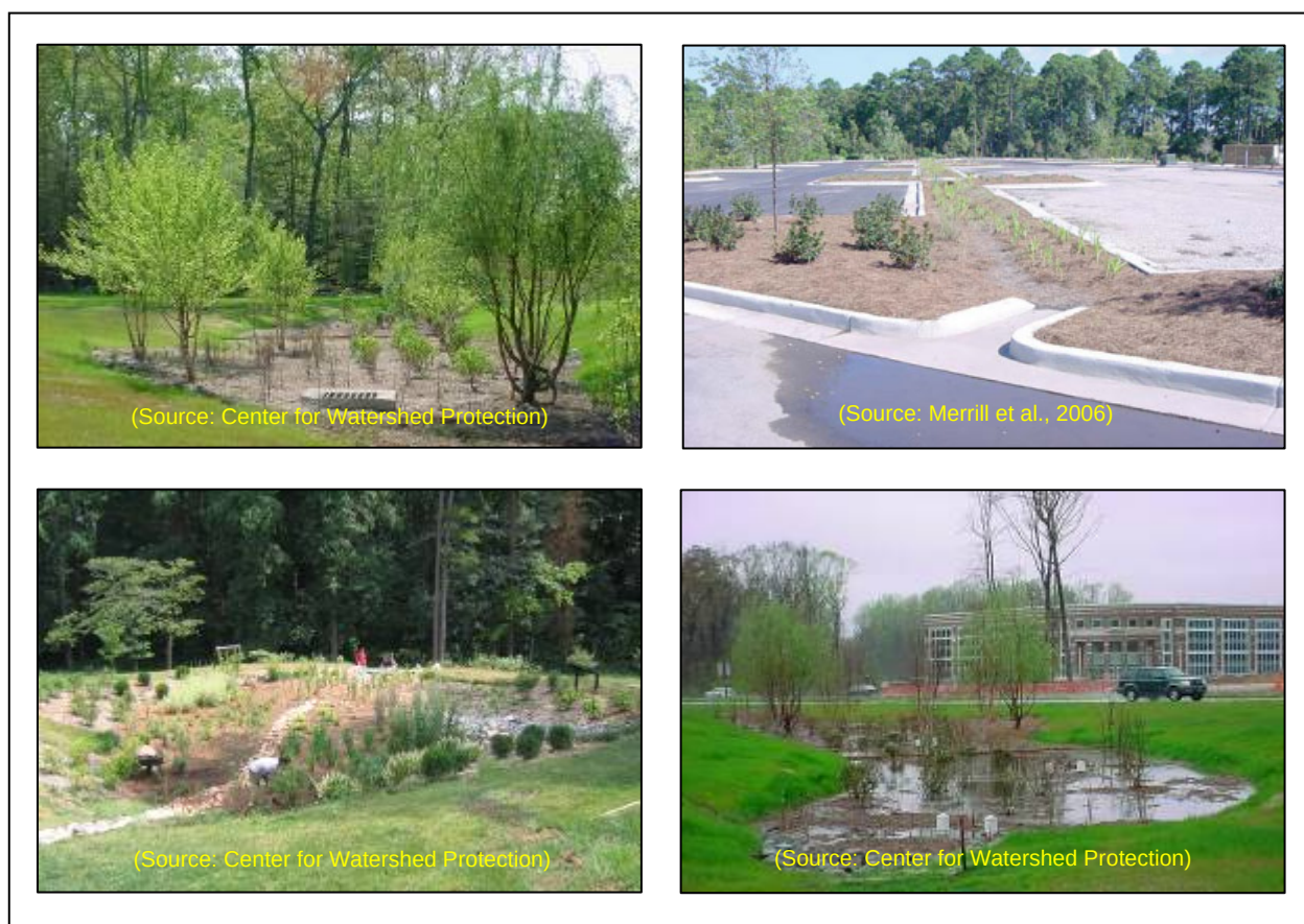
Figure 7.43: Various Bioretention Areas
