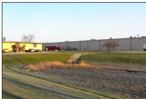
Figure 8.6: Dry Detention Basin Used to Provide Water Quantity Management
