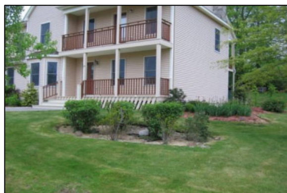
Figure 6.13: Rain Garden Used to “Receive” Stormwater Runoff (Source: Center for Watershed Protection)
