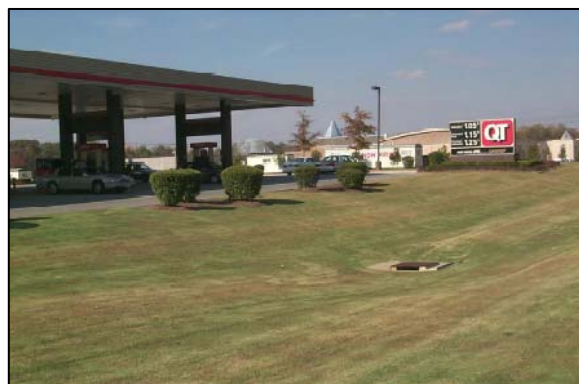
Figure 7.31: Filter Strip Around the Perimeter of a Parking Lot
