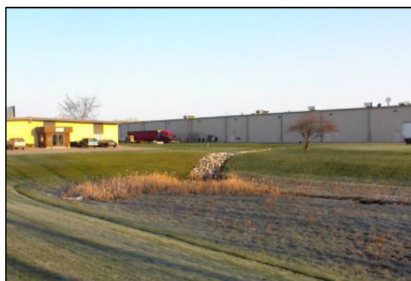
Figure 6.20: Dry Detention Basin Used to Provide Water Quantity Management
