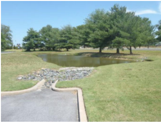
Figure 4. 1. Wet pond with weir outlet structure to road ditch
