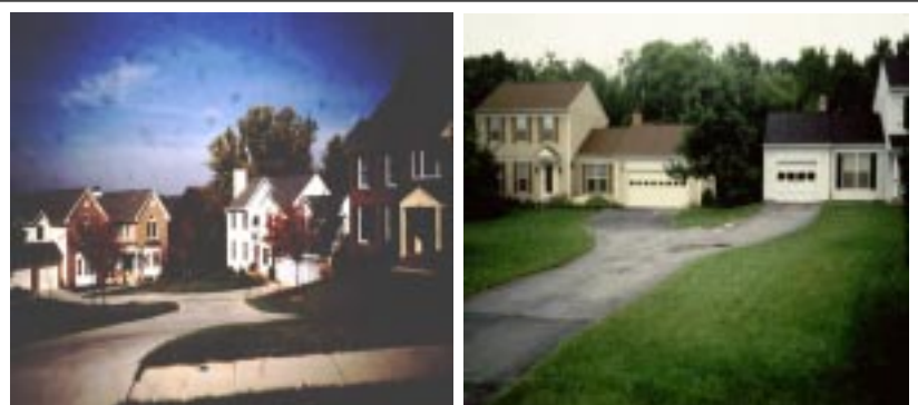
Figure 9: Examples of Different Types of Shared Driveways Shared driveways can help reduce the amount of impervious cover created for parking.
