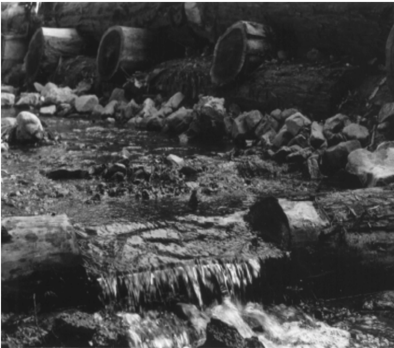
Figure 5: Notched Log Checkdam
