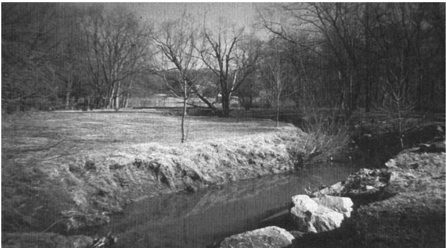
Figure 2: Before Restoration, the Site Was Characterized by Actively Sloughing, Vertical Banks
