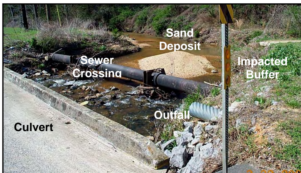
Figure B.1: The STREAM WATCHER protocol is designed to assess overall conditions and potential restoration opportunities in small urban streams. Information is collected on condition of outfalls, riparian buffers, and other impacts as shown here.
