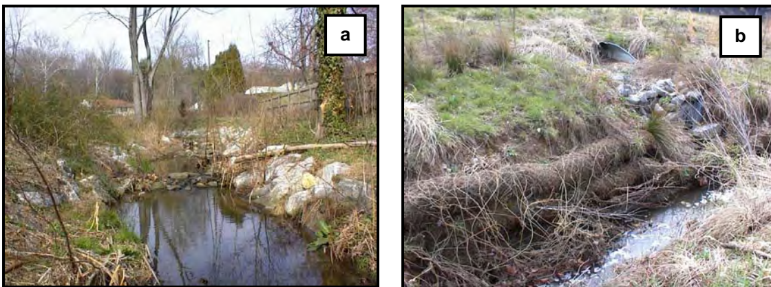
Figure B.11: Bank stabilization practices can be rigid or soft. Panel a shows an example of the use of rip rap to restore eroded section of stream; Panel b shows the mixed use of coir fiber logs and rip rap to stabilize outfall and repair adjacent stream bank.
