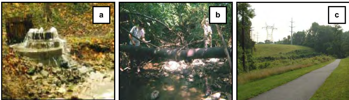
Figure B.18: Common utility-related impacts you may observe include sewer overflows (panel a), damaged and leaking pipe crossings (panel b), or power line rights-of-way interrupting the stream buffer (panel c).
