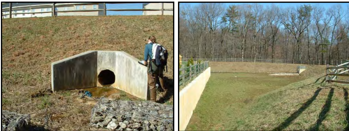
Figure B.8: When assessing an outfall, you may want to take a quick trip up-pipe to determine if the discharge is controlled by a storm water facility. In this case, the outfall is the discharge point for a dry pond. Dry ponds do little for water quality and are therefore good candidates for storm water retrofits.
