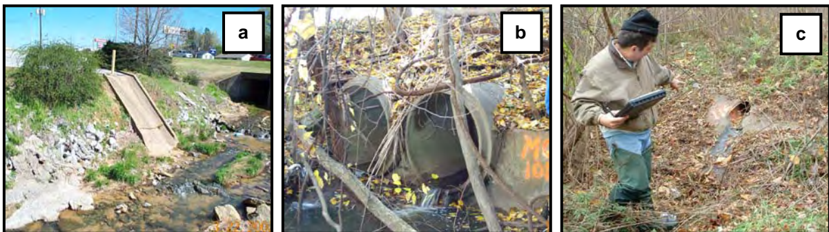
Figure B.3: Storm water outfalls come in a variety of shapes and sizes. For example, not all outfalls will be closed pipes, such as the open channel draining the corner of a commercial parking lot (panel a). Some outfalls may be single or double concrete pipes draining directly to the stream (panel b), while others may be quite small, such as the six-inch diameter pipes discharging into the buffer in panel c.
