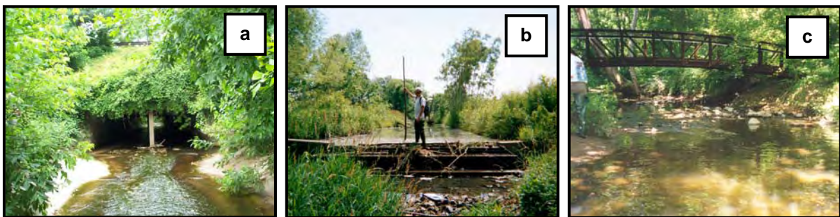
Figure B.20: Roadways (panel a), dams (panel b), and pedestrian bridges (panel c) are structured crossings that you may observe. You should assess all crossings that have a direct impact on the stream. Structures like the one shown in panel c that do not have a significant impact should not be assessed.
