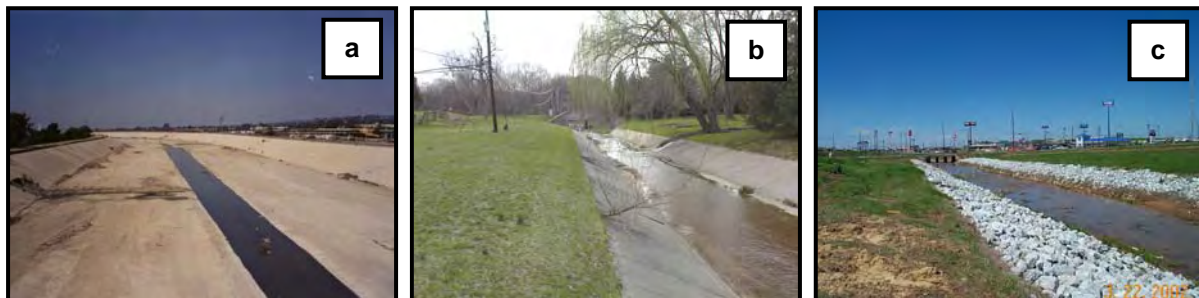
Figure B.24: Various types of channelized streams include a concrete channel and flood plain (panel a), a concrete-lined channel (panel b), and an armored stream segment (panel c).
