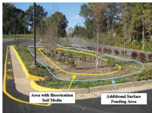
Figure 1. Adaptation of bioretention facility. Additional surface ponding area can be incorporated (light blue line) while the surface area and volume of soil media remain the same (yellow line). The photo shows a conceptual approach of how the design adaptation may be accomplished. Photo courtesy of: Williamsburg Environmental Group, Inc.
