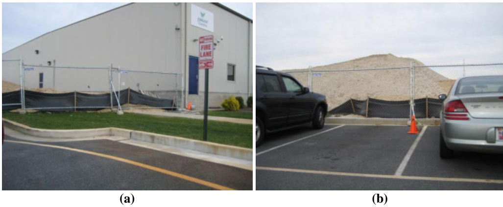
Figure 4.26. HSI_31 (a) and (b) Poor erosion and sediment control (ESC) practices at Jubilant Cadista.
