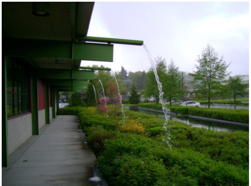
Figure 5. Downspouts at the BES lab disconnected from the combined sewer system and directed into infiltration swales next to the Willamette River (Printed with permission ©2013 Environmental Services, City of Portland, OR)
