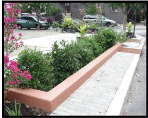
Figure 15: Infiltration trench at Clark Park.
