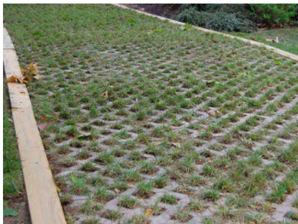
Montgomery County's restoration plan focuses heavily on installing stormwater retrofits, such as this permeable pavement, on existing developed land (Source: Chesapeake Bay Program)
