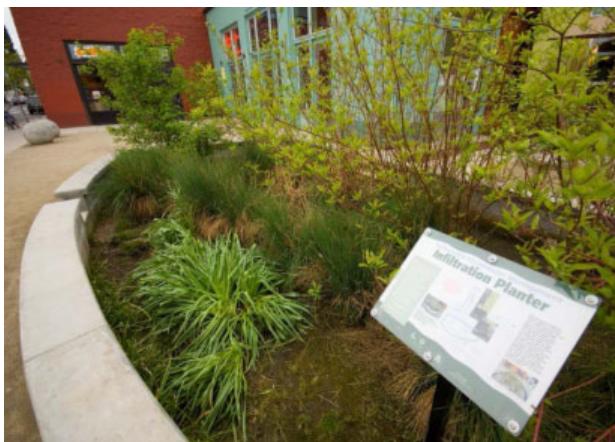
In Prince George's County, infiltration practices, such as this planter, will be installed to treat more than 5,400 acres of land (Source: Radcliffe Dacanay).
