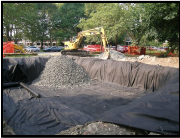
Figure 14: Stormwater trench at Columbus Square.
