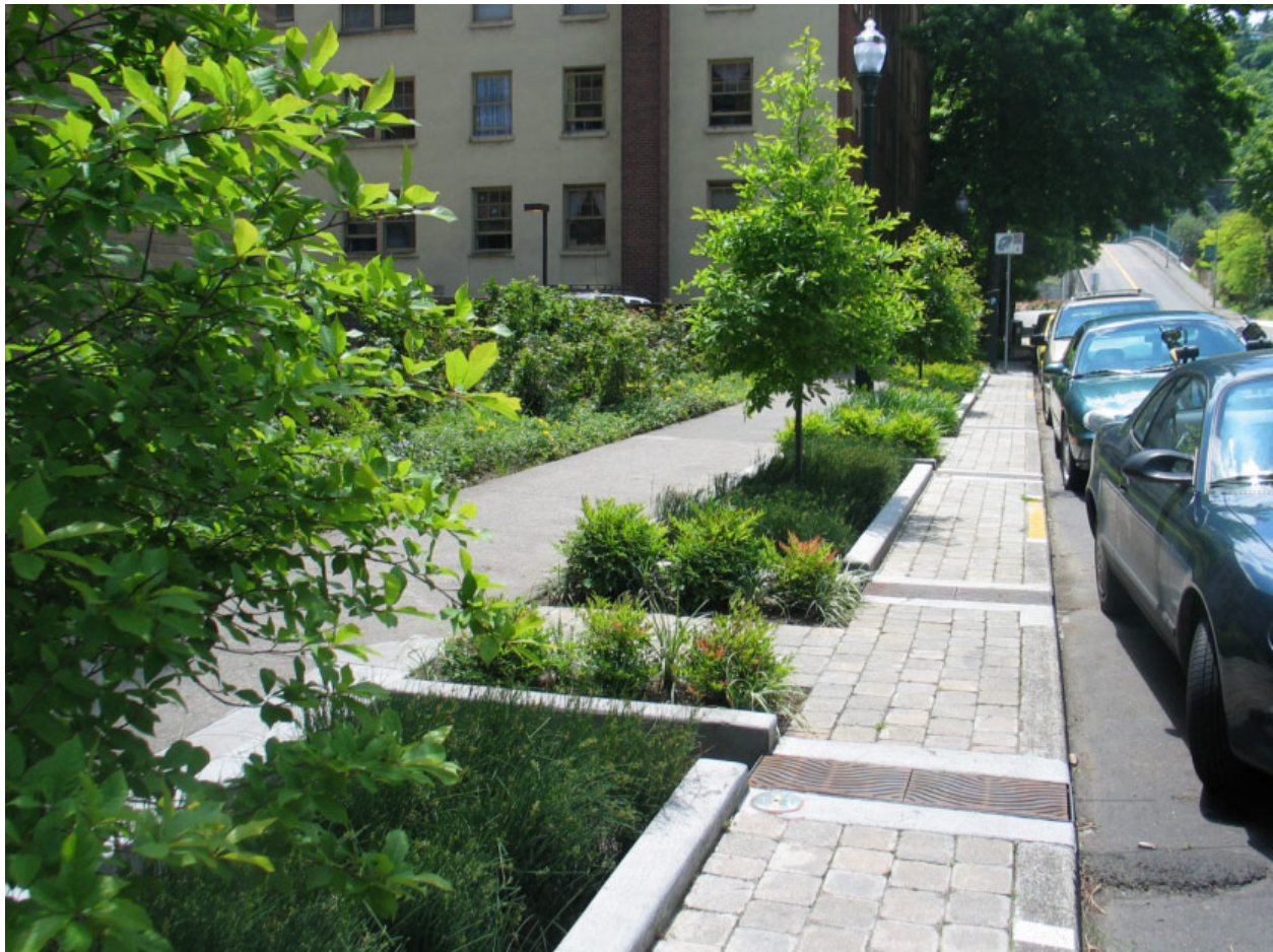
Figure 6. The SW 12th Avenue Green Street at SW 12th and Montgomery on the Portland State University campus utilizes a series of landscaped stormwater planters designed to capture and infiltrate approximately 8,000 square feet of street runoff. This innovative streetscape project effectively manages street runoff while still maintaining strong pedestrian circulation and on-street parking. Built in summer 2005, this street retrofit project demonstrates how both new and existing streets in downtown or highly urbanized areas can be designed to provide direct environmental benefits and be aesthetically integrated into the urban streetscape. This green street project is effective and functional, and it also successfully integrates landscaped stormwater planters into the urban fabric (Printed with permission ©2013 Environmental Services, City of Portland, OR)
