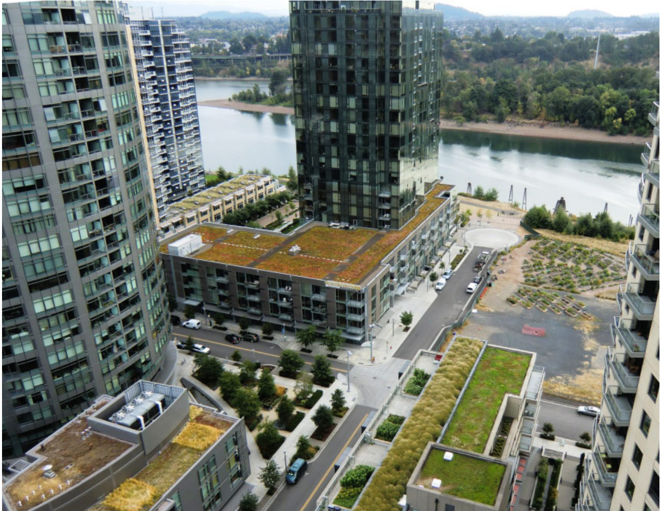
Figure 13. Ecoroofs at Portland's south waterfront neighborhood (Printed with permission ©2013 Environmental Services, City of Portland, OR)
