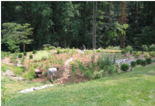
Howard County plans to install bioretention practices like this one that will treat more than 2,000 acres of land in the county (Source: Center for Watershed Protection)
