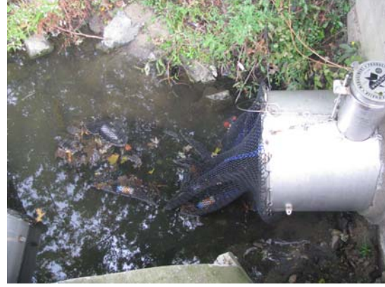
b) Glenwood Circular is a 36-inch outfall.
