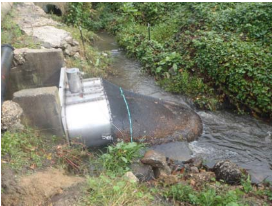
c) Earle 48 is a 48-inch outfall.
