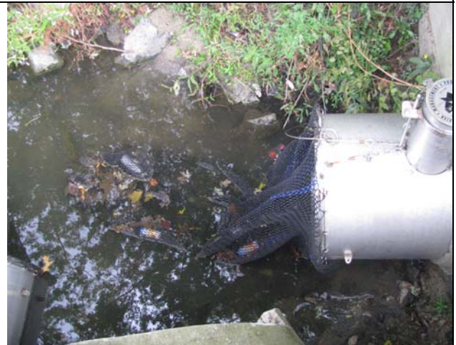
c) Glenwood Circular outfall is 36 inch.
