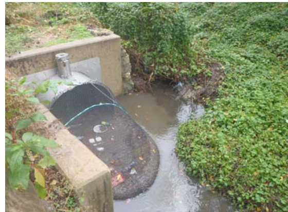
d) Earle 60 is a 60-inch outfall.
