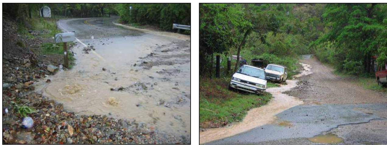
Figure 3. Route 108 inlet blockage/backup (left); and Gerda Marsh Rd. runoff (right)
