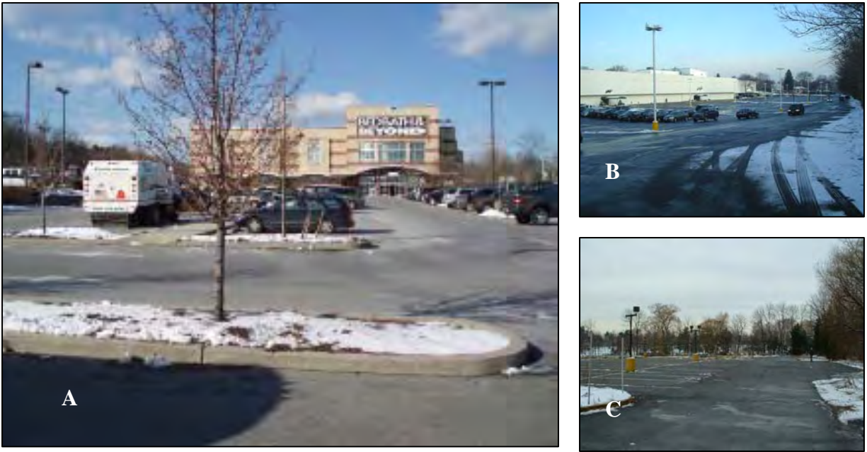
Figure 3-24: Parking lots at commercial shopping centers and businesses offer many opportunities to collect and treat stormwater runoff. (A) This shared parking lot at the Bed Bath & Beyond in Manhattan Park Brook (site ID MP-R2) is a potential candidate for underground sand filters. (B) The Lord and Taylor in Bronx River Middle Direct Drainage (site ID BRM R2) and (C) Frank's Nursery in Grassy Sprain Brook (site ID GSB-R1) offer bioretention, porous pavement and vegetative swales options.
