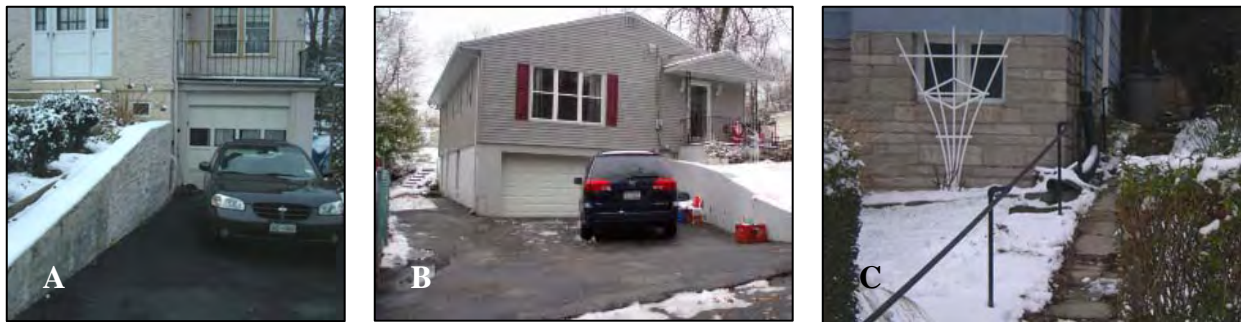
Figure 3-14: Opportunities for downspout disconnection in residential areas are plentiful. (A) shows a downspout directly connected to the storm drain system or to outlets on the street curb (B) shows a downspout draining onto driveway, which may subsequently drain to a pervious area or to the storm inlets on the street. (C) Shows a diverted downspout into a lawn area or landscape feature, which is preferable where feasible.
