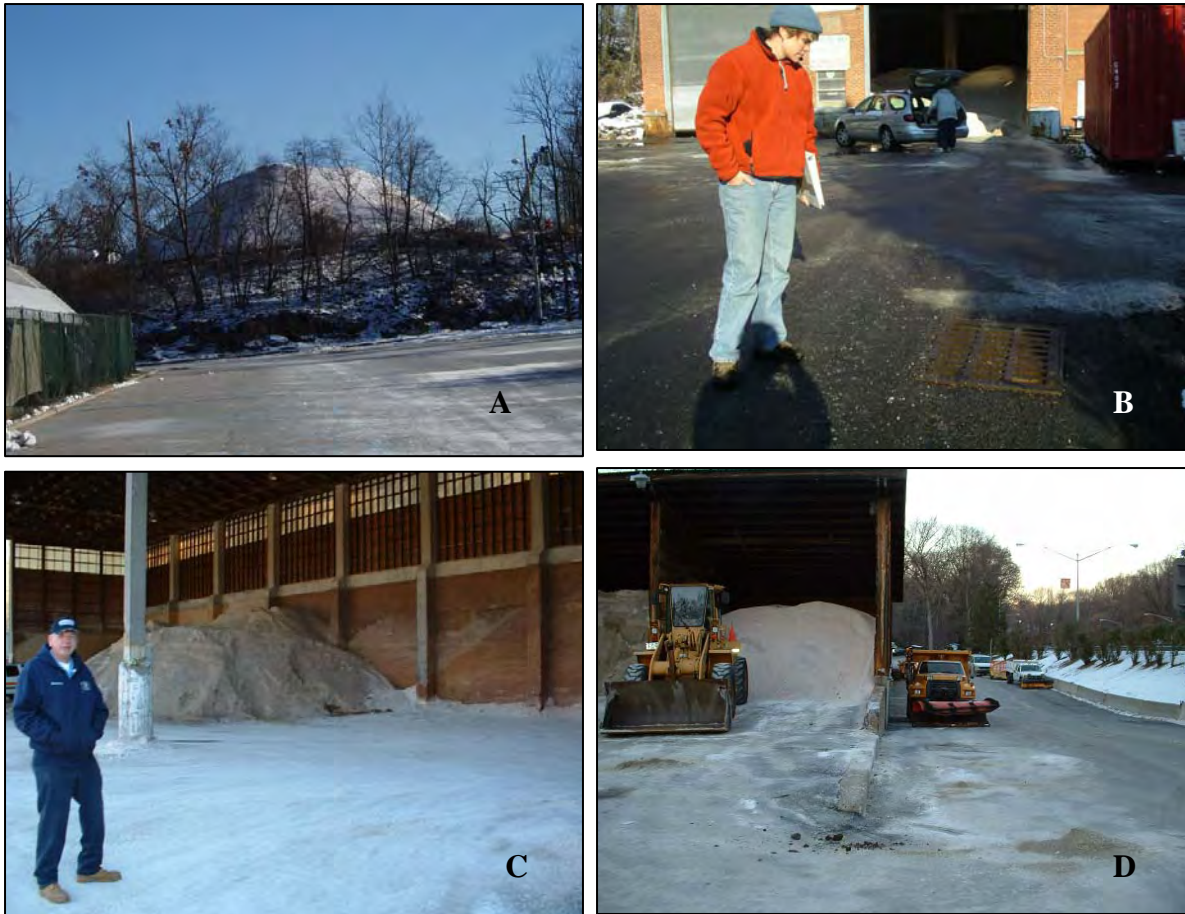
Figure 3-12: Salt storage practices ranged from (A) uncovered stockpiles in Yonkers, to covered storage areas that were (B and D) directly connected to storm drains in Eastchester and County Reservation Yard, or (C) were sloped to help contain salt in Greenburgh.
