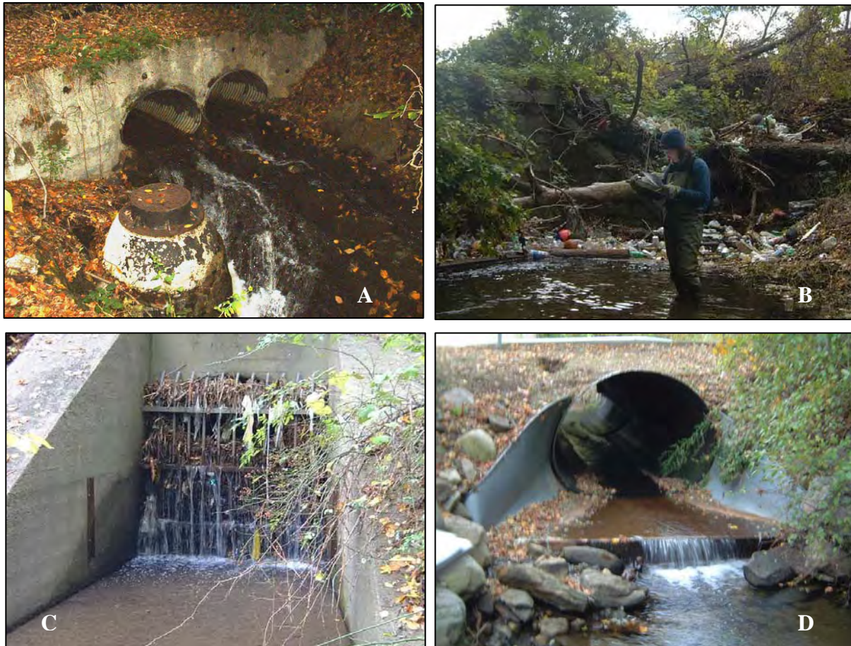
Figure 3-7: Field teams noted potential problems with utility crossings (A), and culverts that required debris or trash removal, such as (B) a debris jam and trash accumulation and (C) a blocked grated culvert in Davis Brook in reach DB-8. (D) Locations of potential fish barriers were also noted like the one here in Davis Brook in reach DB-2.
