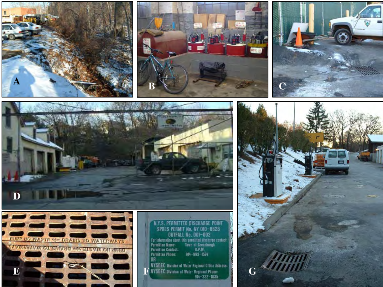
Figure 3-10: Municipal maintenance facilities were confirmed hotspots, though good practices were observed. Specific observations include: (A) stream and wetland encroachment; (B) secondary containment; (C and D) evidence of polluted drainage to storm drains; (E) drain stenciling; (F) posting of signage; (G) fueling islands draining directly to storm drains.
