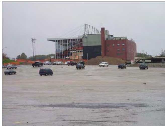
Figure 3-11: The racetrack in Yonkers provided stormwater retrofit, pollution prevention, and erosion and sediment control opportunities during construction.
