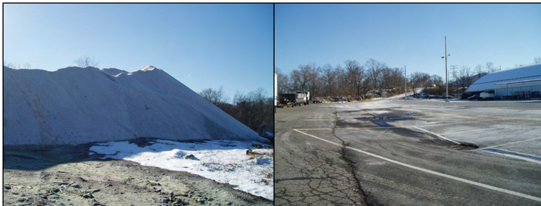
Figure 7-4: Salt storage area in City of Yonkers
