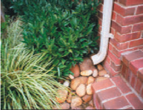
Figure 6.7: A disconnected downspout in Rivergate.
